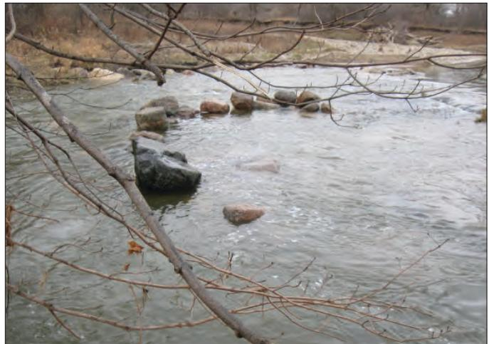
*A close-up of the j-hook stabilization method utilized in the bank restoration project on the Redwood River near Lynd, Lyon County. J-hooks are positioned in such a way to provide a deep pool habitat at the point of the hook while redirecting stream flow to inhibit bank erosion downstream.*
