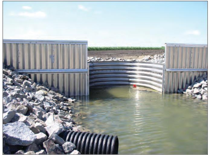
*Meeker County, six foot aluminum drop structure at the head of a private ditch to control gully erosion and bank erosion.*
