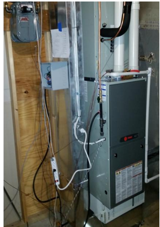
Figure 3. Ducted Whole House Cold-Climate Air-Source Heat Pump, which Includes an Outdoor Condenser unit (left) that is connected to an Evaporator Coil installed in the Ductwork of the Forced-Air Furnace Inside the Home (right) (Pictures courtesy of the Center for Energy and Environment).
