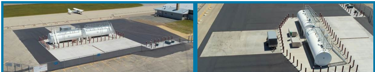
The Fuel System at Crystal Airport Opened in July 2020
