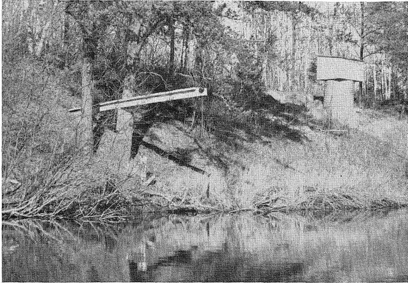
**EQUIPMENT** for checking surface water fluctuations include the recording well and shelter at the right and the outside return gage at the left. This scene is on the Sturgeon river near Chisholm.
