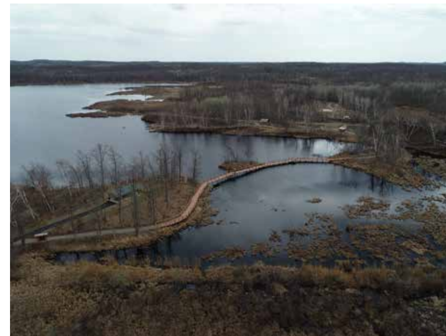
Crow Wing County Milford Mine Boardwalk
