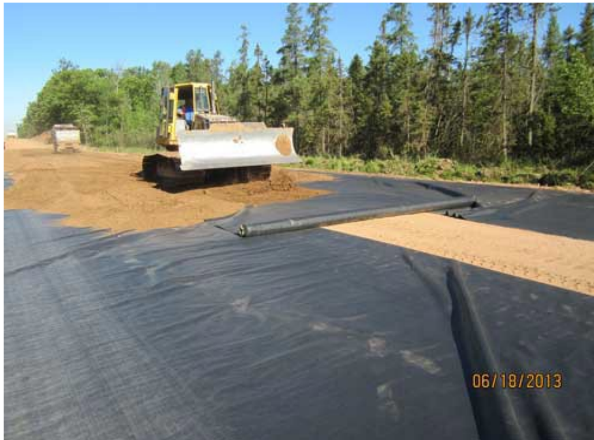
Figure 14: Construction of the nine-ton road surface on County Road 132
