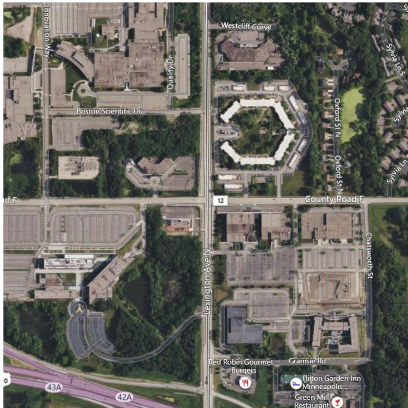
Figure 19: Lexington Ave and County Road F intersection improvement
