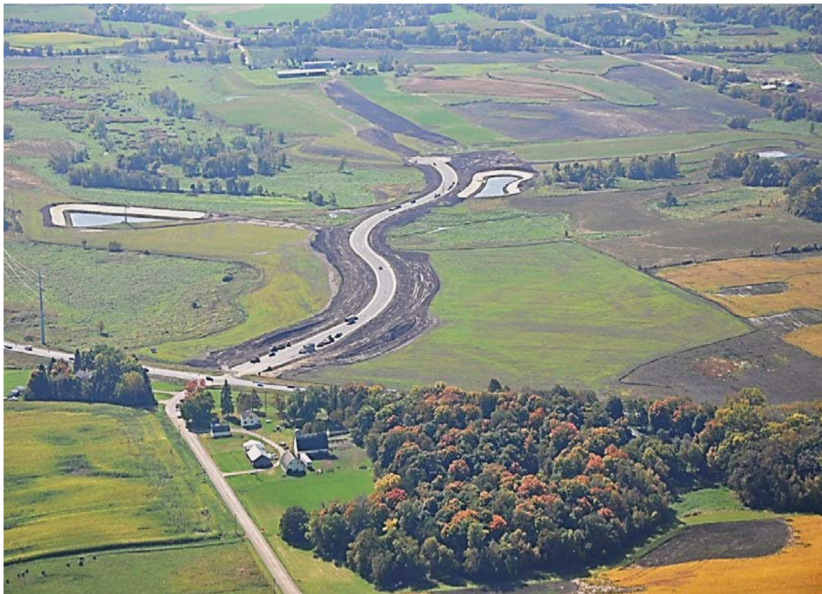
Figure 12: Delano Business Park access road
