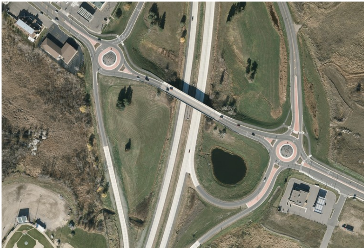
Figure 11: State Highway 10 and County Rd 3 Interchange
