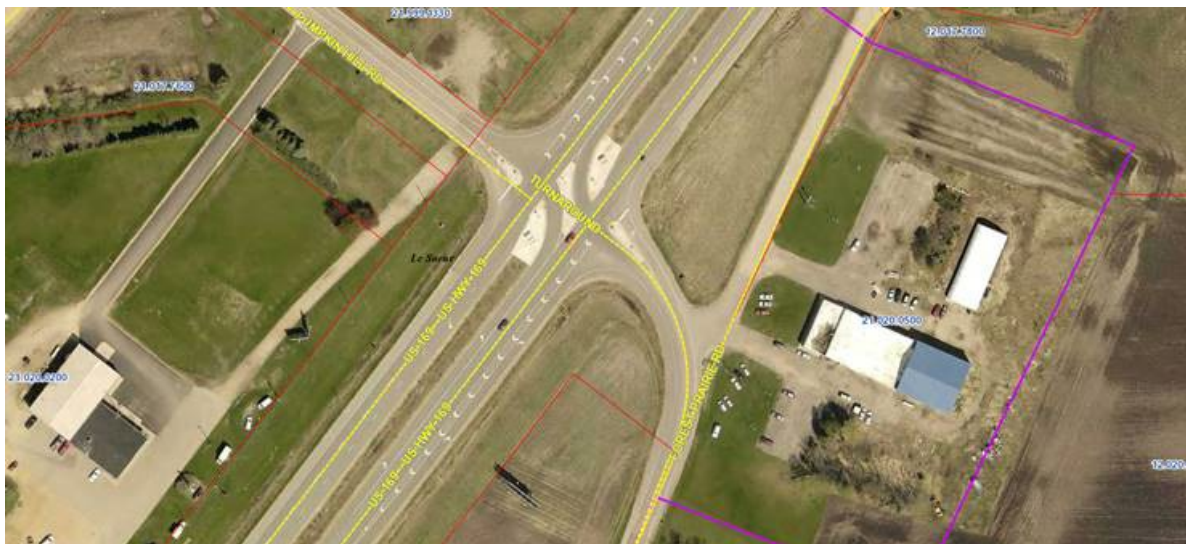
Figure 25: A Portion of the completed project; Le Sueur TH 169
