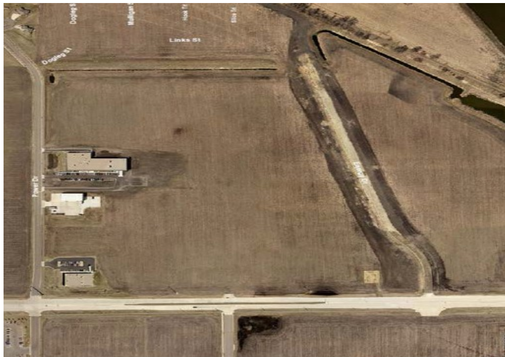
Figure 10: Eastwood Industrial Energy Park access road
