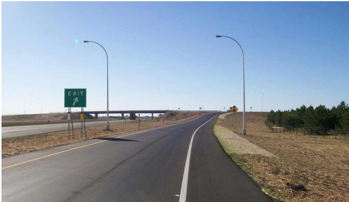
Figure 1: Exit ramp from TH 10 to CSAH 34
