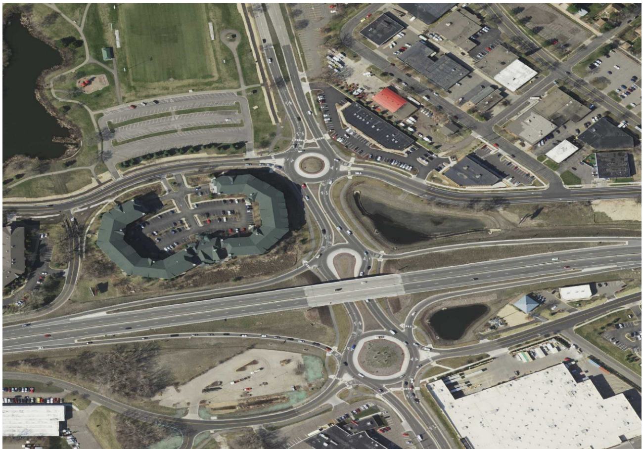
Figure 21: Completed TH 7 and Louisiana Ave Interchange
