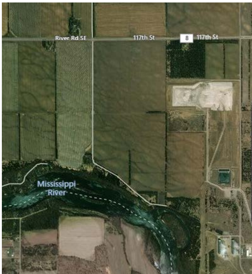
Figure 51: Becker Business Park
