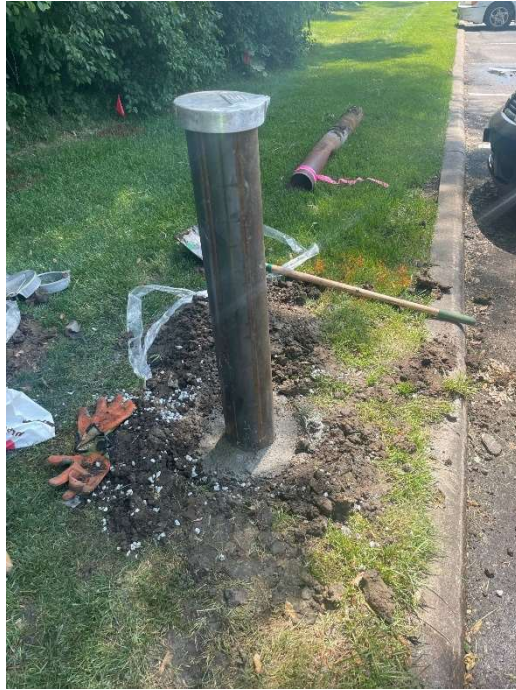
Photo 5: Complete replacement of PSG-03 facing south
