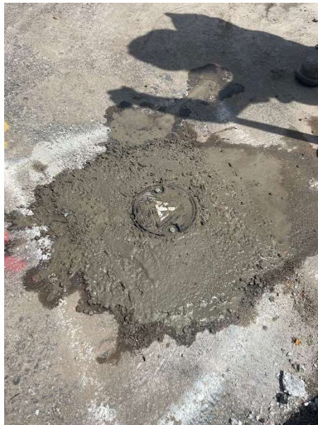
Photo 6: Completed replacement of PSG-06 vault
