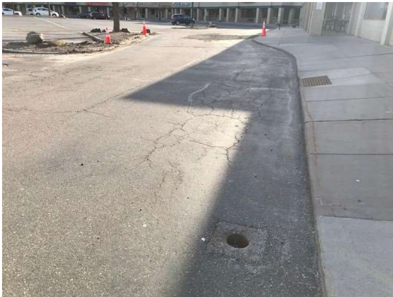
Photo 2: PSG-06 vault in foreground facing east
