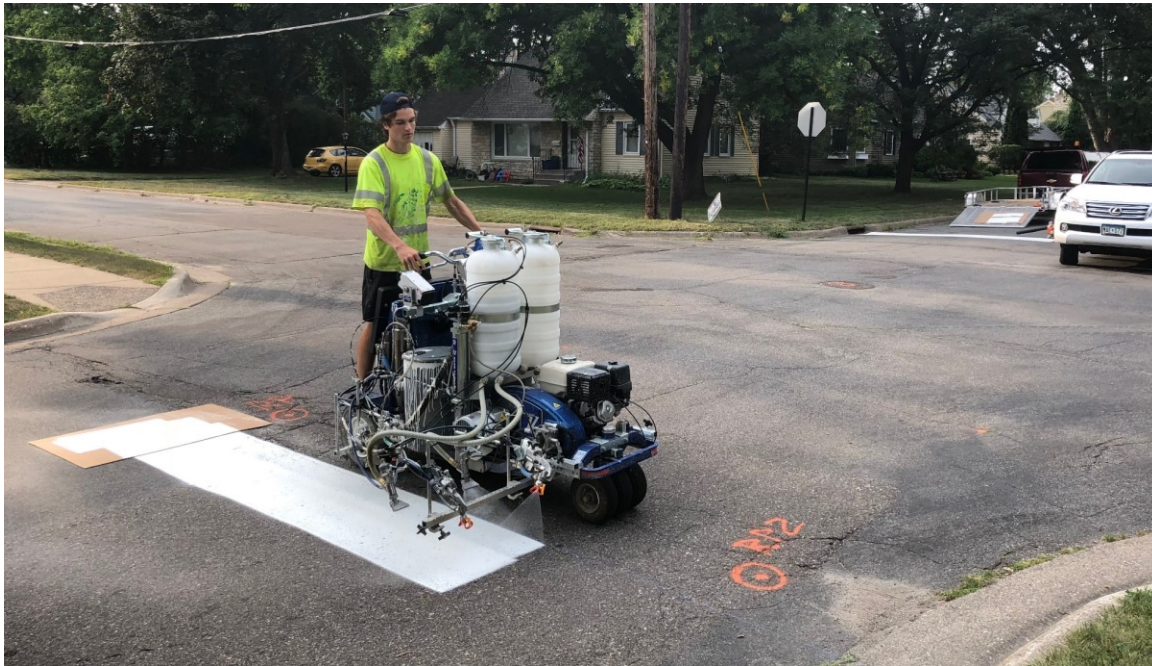
Figure 3.3 Painting of stop lines
