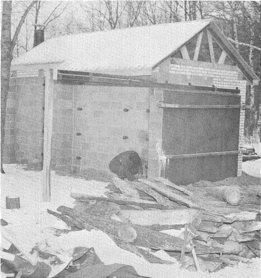
KILN ERECTED for tests in charcoal production.
