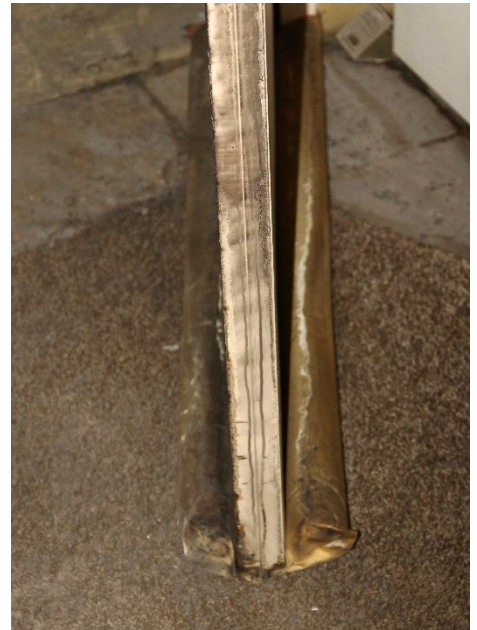
Figure 9: Seal under door of adjacent apartment
