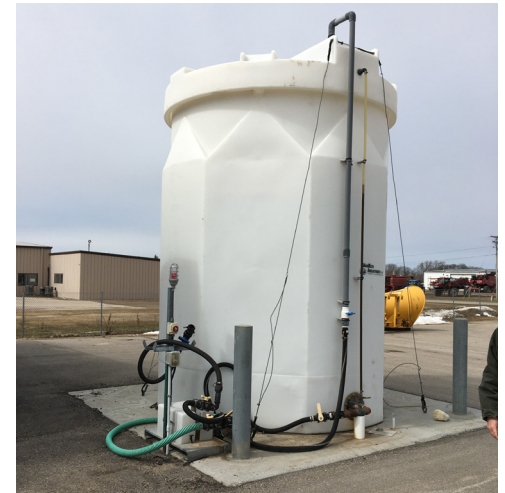
District 2 storage tank for salt slurry
