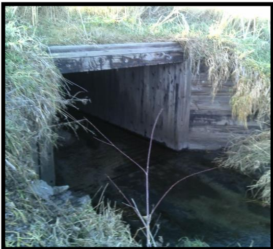
Figure5 – Wooden culvert on Fillmore County Highway 1
