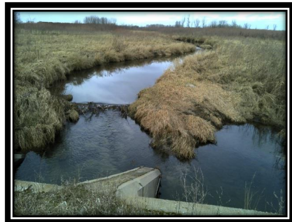
Figure 2 - Poorly Aligned Culvert on Pine Creek.
