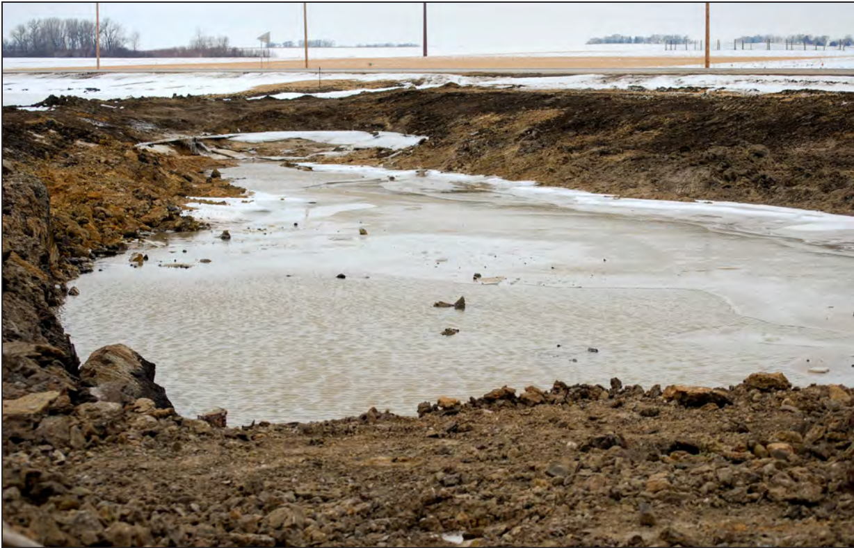
A tributary to the South Branch Vermillion River will be diverted around a constructed wetland in Castle Rock Township while the plants take hold. The experimental nitrate treatment is slated to go online in 2019. Final ground work is scheduled for this spring. Photo Credit: BWSR
