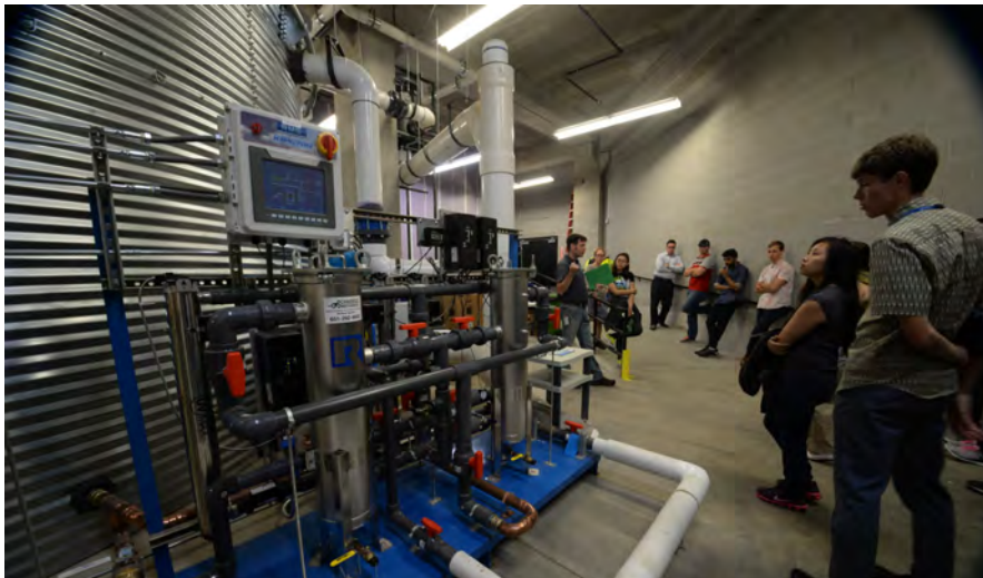
Figure 15. Stormwater reuse is showcased on tours of the cistern that holds rainwater captured from the roof of Metro Transit's Green Line Operations and Maintenance Facility, for use at CHS Field.
