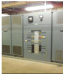
ANOKA-RAMSEY: electrical panels
