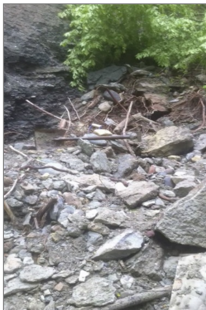
Figure 63. Landslide in Lilydale in 2013
