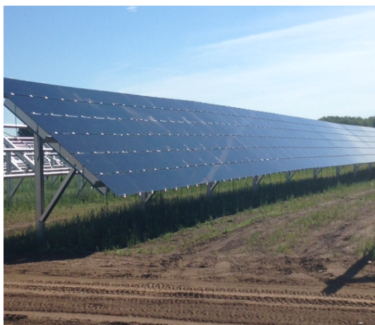
First Solar thin film modules were selected for the 10-megawatt solar photovoltaic power plant. These advanced thin film modules have a demonstrated performance advantage over conventional crystalline silicon of up to 10% more energy production each year. Source: MN National Guard Public Affairs Office
