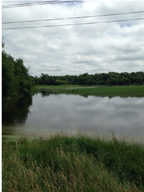
Constructed wetland in foreground provides additional water storage capacity to reduce field flooding, visible in background. Photo: Dustin Benes, Martin County SWCD.
