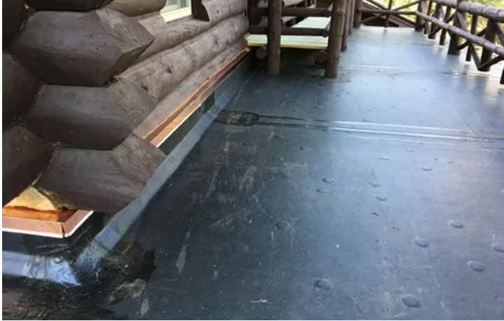
Photo 8: Itasca State Park Douglas Lodge roof membrane in poor condition replaced in 2018.
