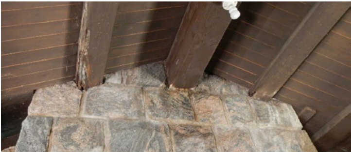
Photo 29: Fort Ridgely State Park Day-use Area shelter—ceiling wood truss rot.
