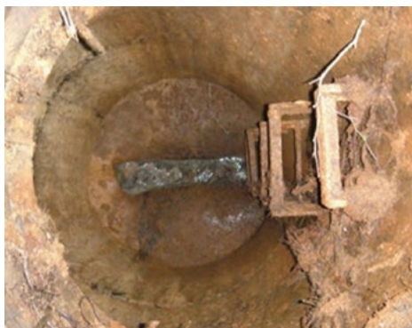
Photo 15: Itasca State Park—manhole in crisis condition.
