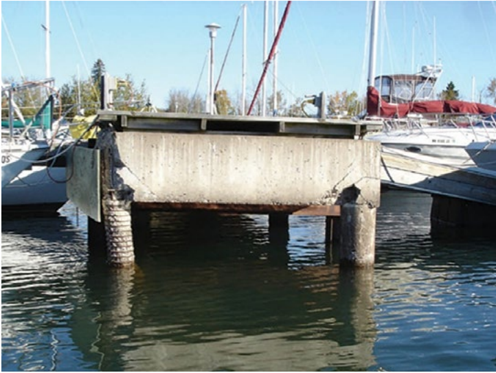
Photo 27: Knife River Marina—failing pier.
