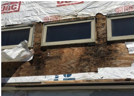
Photo 4: Windom Co-located Office exterior water damage.
