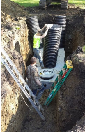
Figure 25. Installation of a typical septic tank and mound drain field, Watonwan County.
