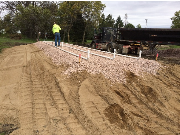
Figure 25. Installation of a typical septic tank and mound drain field, Watonwan County.
