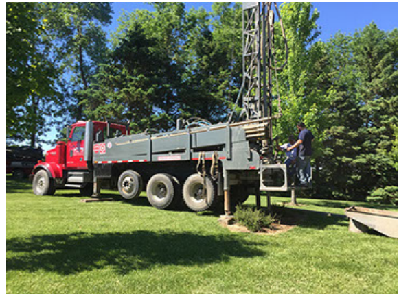
Figure 29. Typical well drilling installation.
