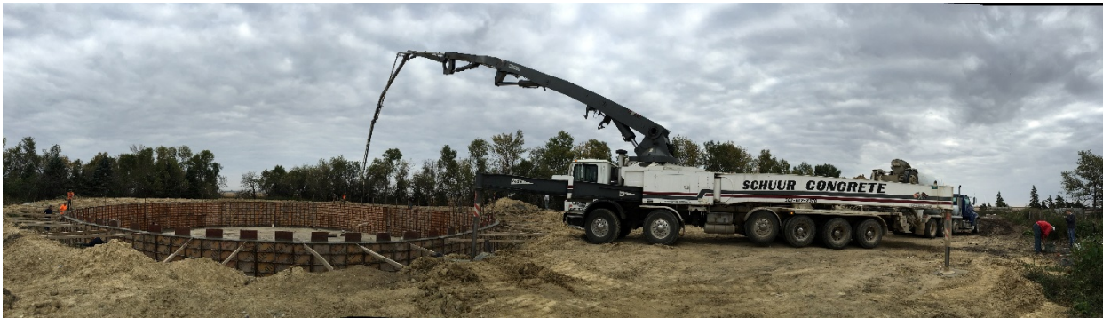
Figure 15. Installation of manure storage structure in Olmsted County.
