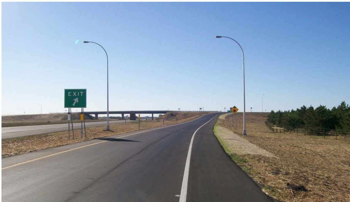
Figure 1: Exit ramp from TH 10 to CSAH 34
