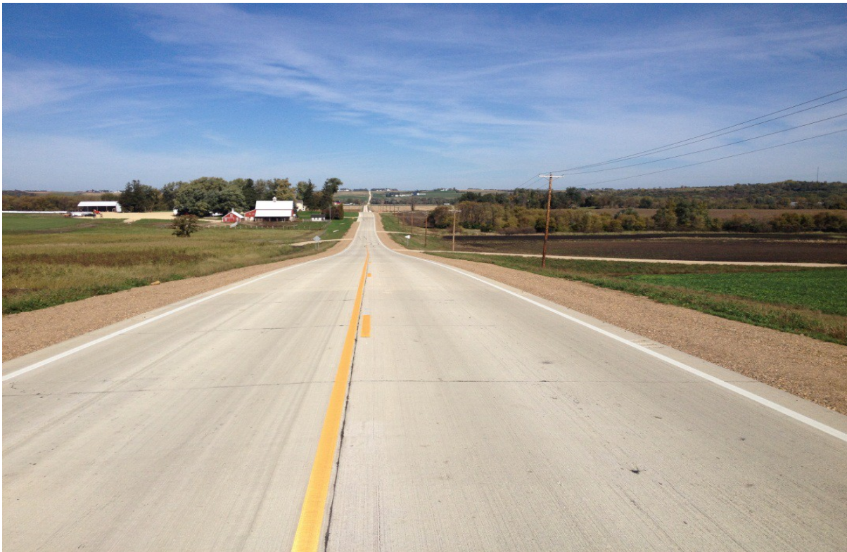
Figure 2: TH 52 project completed in conjunction with the Versa Cold expansion
