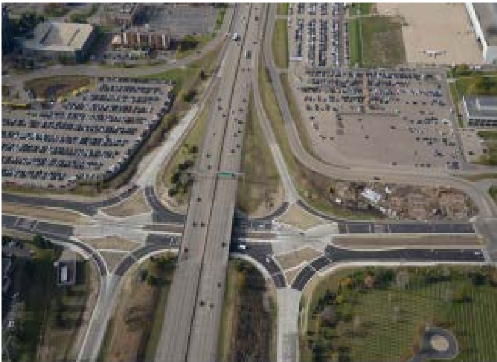
Figure 9: Bird's eye view of the I-494 34th Ave Interchange
