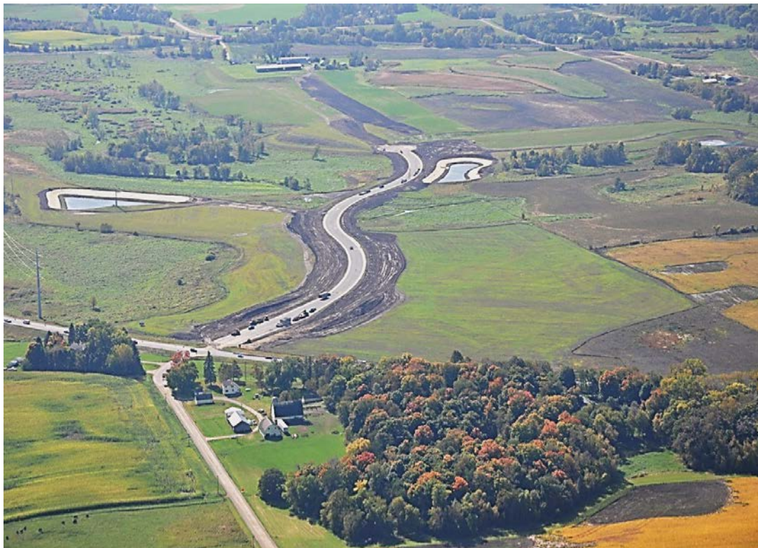
Figure 12: Delano Business Park access road
