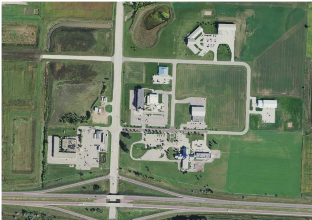
Figure 3: Trunk Highway 59 Infrastructure Improvements
