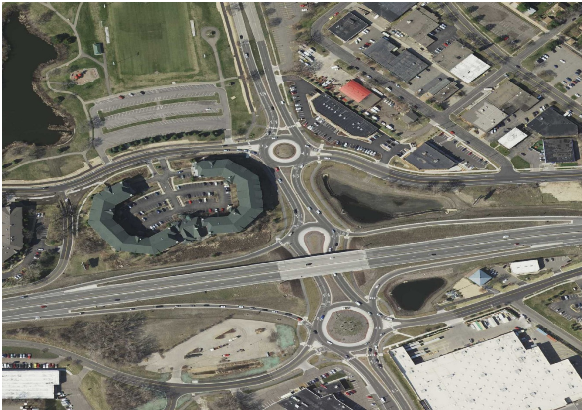
Figure 21: Completed TH 7 and Louisiana Ave Interchange
