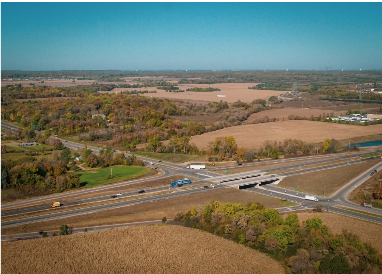
Figure 28: Ariel View of TH 52-CSAH 42 Interchange reconstruction, Dakota County
