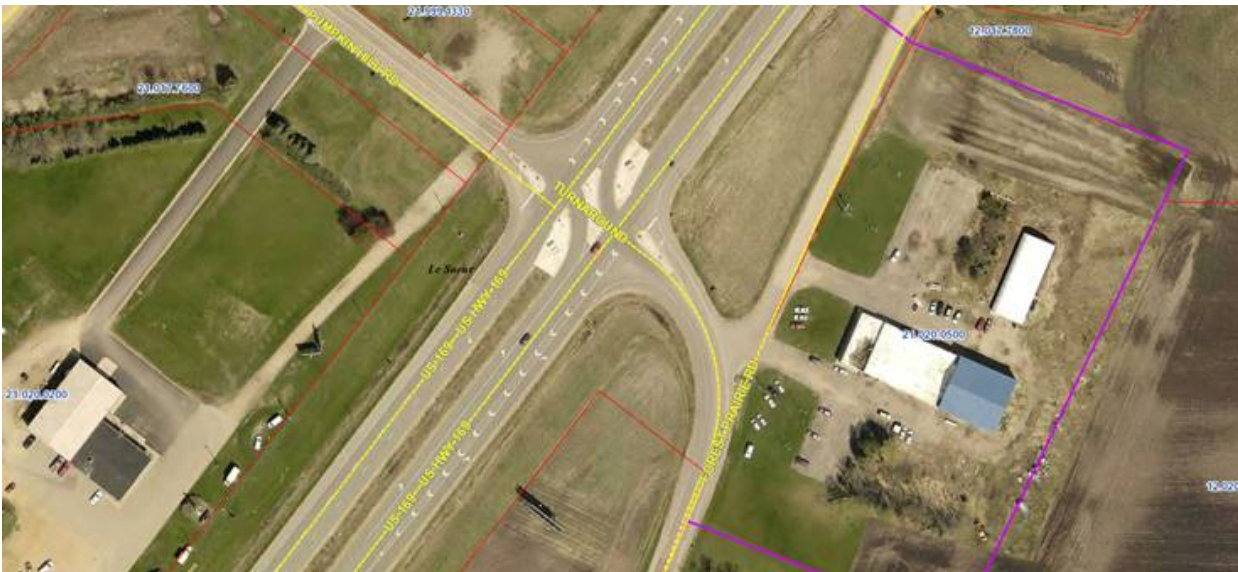
Figure 25: A Portion of the completed project; Le Sueur TH 169
