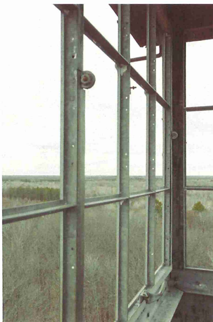
Sash without glass – St. Croix Fire Lookout Tower. The sash is stamped “Fenestra.” It was made by Detroit Steel Products Company, a common supplier of fire tower windows (see the Fenestra trade catalog in this report’s References).
