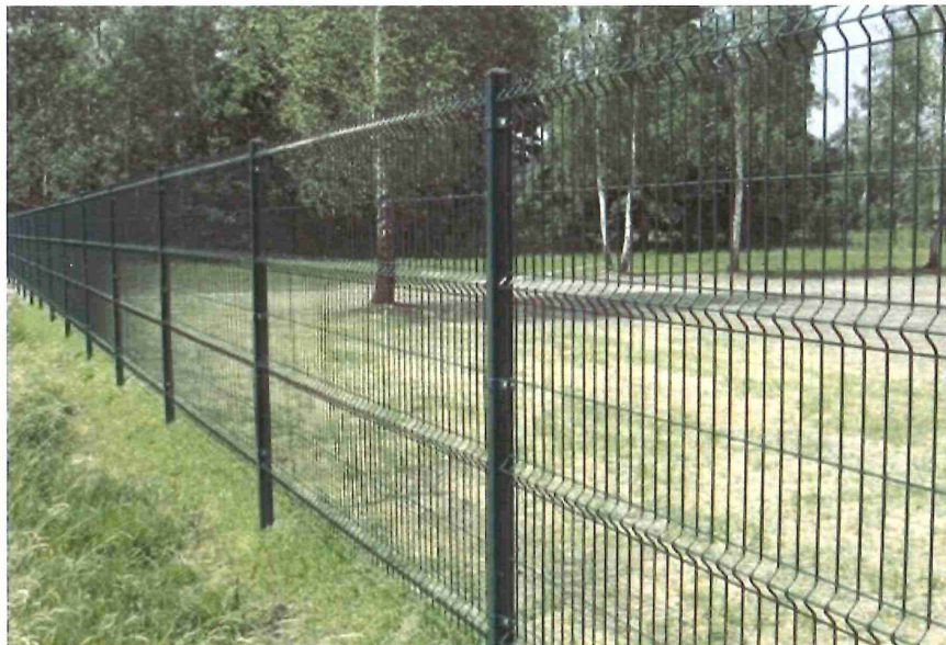
Simple wire fence with metal posts. The mesh has horizontal crimping for added strength so a top horizontal rail is not needed (internet photo)
