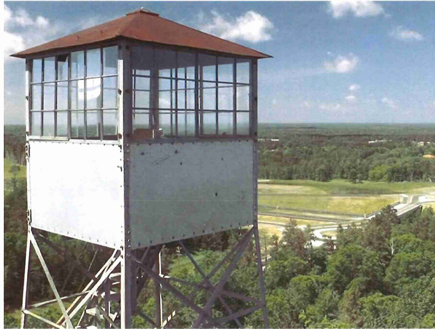
Reglazed sash – Pequot Fire Lookout Tower (photo by Travis Grimler, Pine and Lakes Echo Journal )
