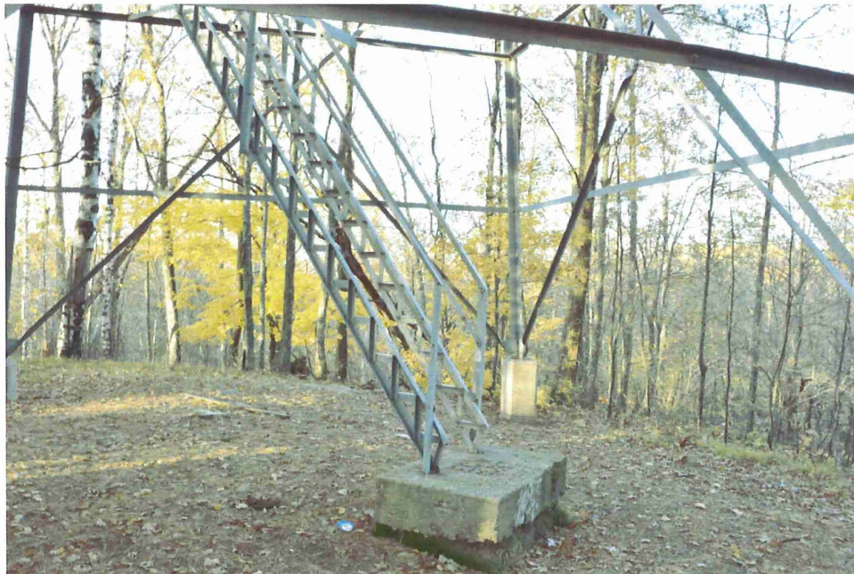
Stair treads removed – Ben Draper Fire Lookout Tower
