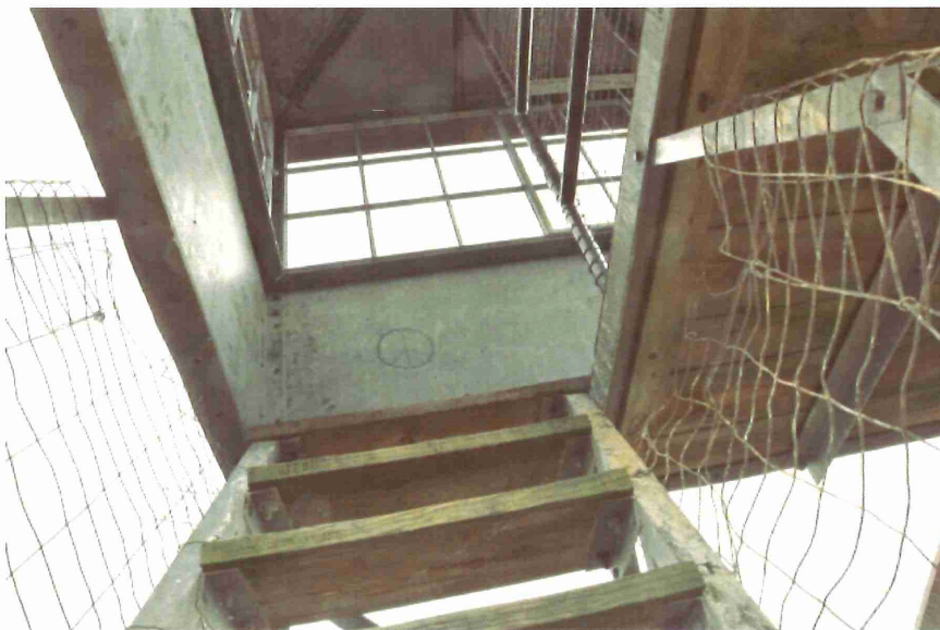
Example of railing with no gap at the cab – St. Croix Fire Lookout Tower
