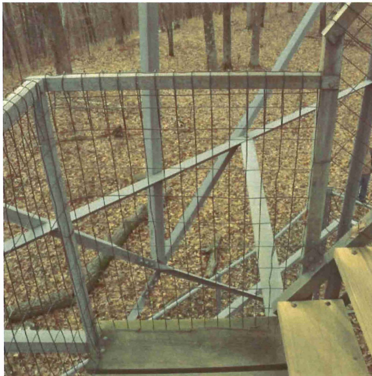
Example of original angle handrail on an Aermotor tower – St. Croix Fire Lookout Tower
