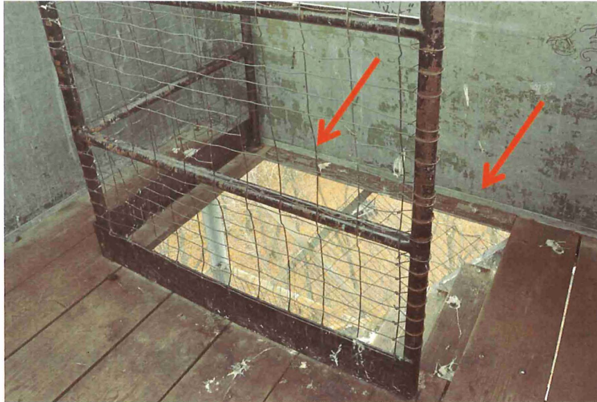
The trap door has been removed but arrows point to the marks left by the hinges – St. Croix Fire Lookout Tower
