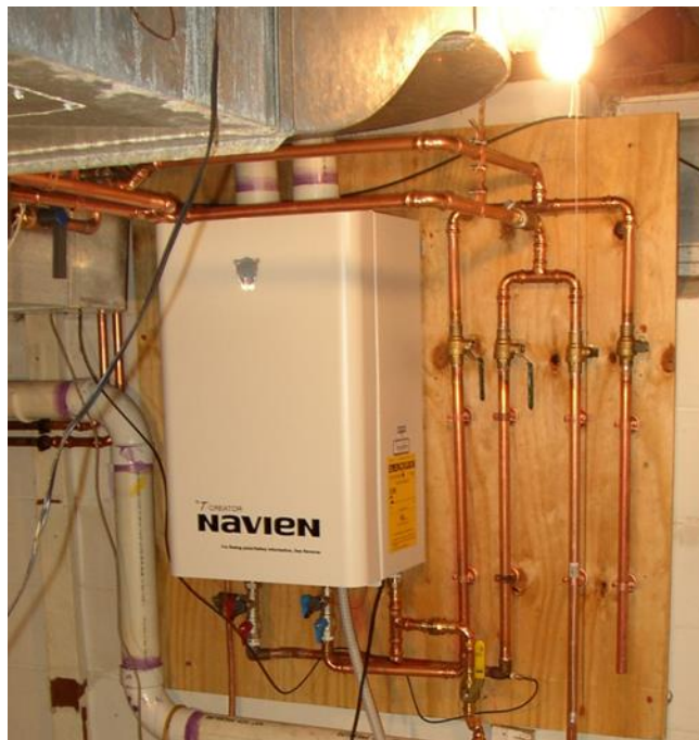
Figure 33. Example of a tankless water heater
