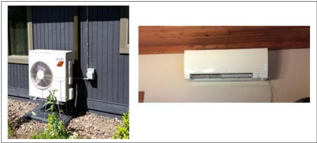
Figure 26. Example of installed cold climate ductless mini-split air-source heat pump.
