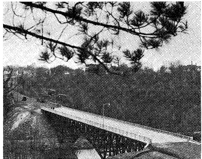
This 400-foot long bridge carries TH 123 over the Kettle River on the east side of Sandstone. The three-span steel arch structure replaced an old four-ton load limit bridge. It was completed in 1948.
