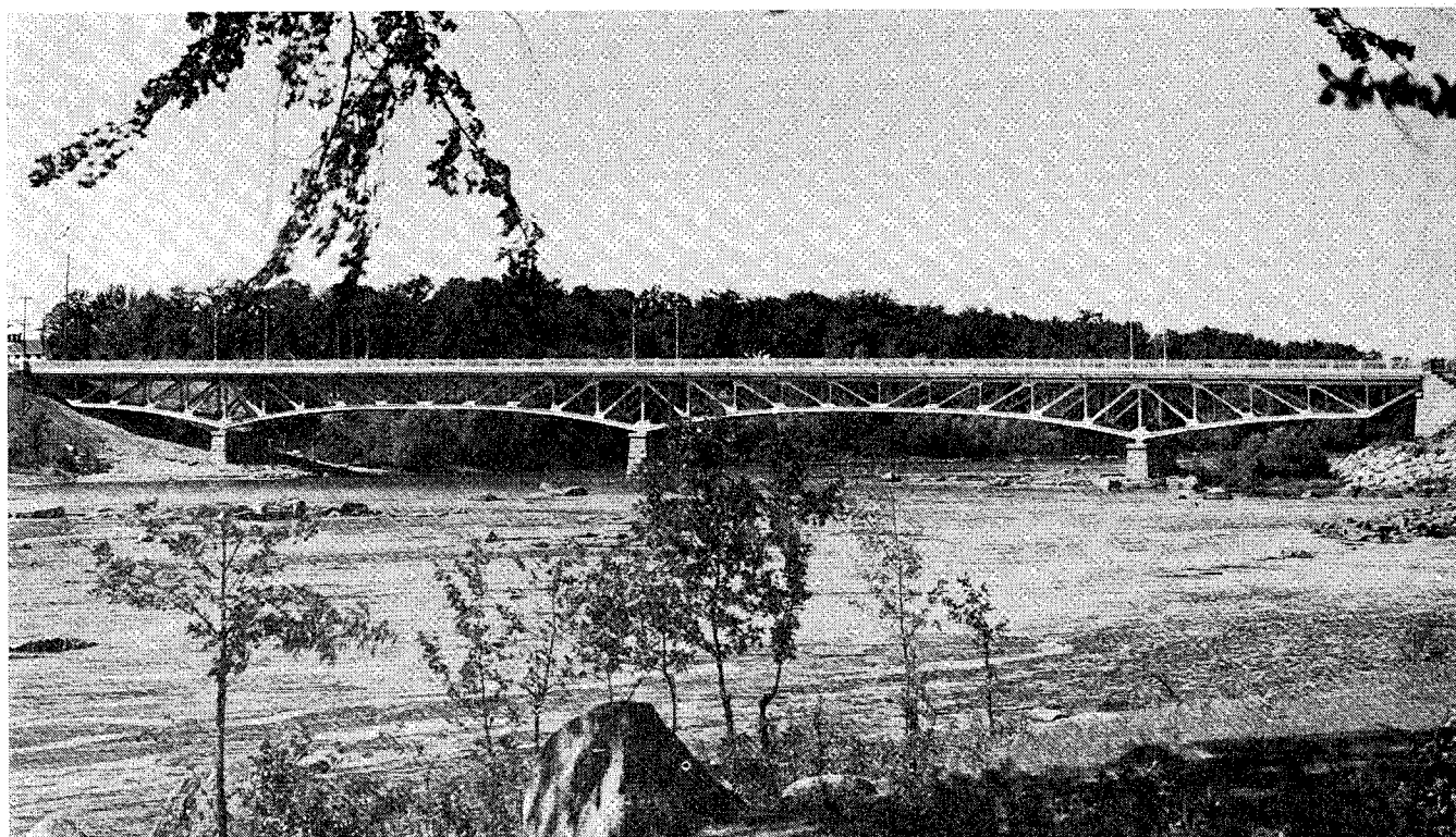
A project of 1947-48 was bridge No. 5947 over the Mississippi River at Sauk Rapids. It is 555 feet long with a 27-foot roadway between curbs and a five-foot pedestrian sidewalk. The cost was $193,600.
