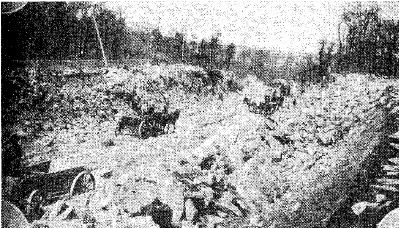
This 1924 photo pictures the construction of TH 44 in Houston County, with horse-drawn dump wagons used in a cut of the rocky terrain.
