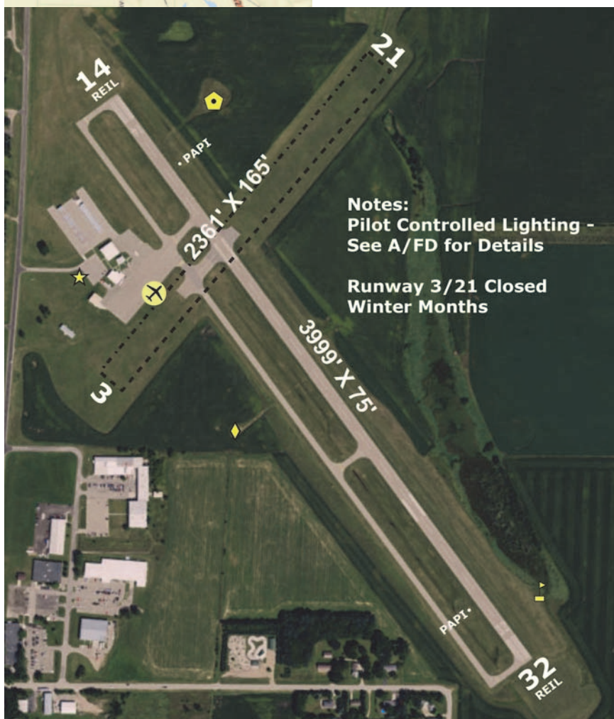
Montevideo-Chippewa County Airport
