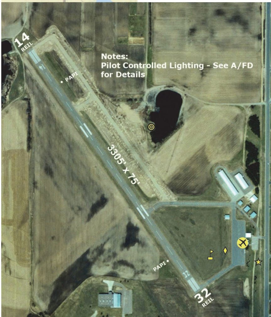
Staples Municipal Airport
