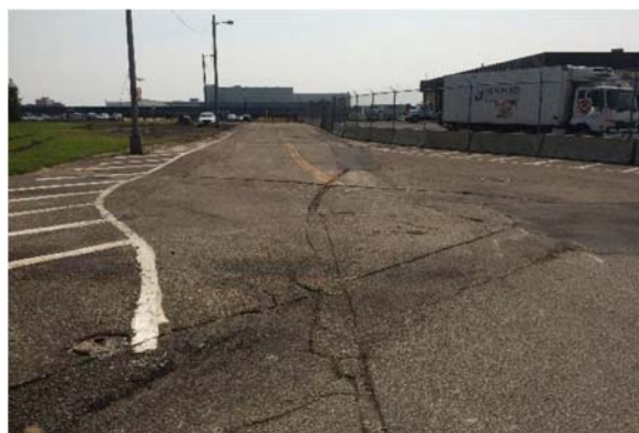
Landside Pavement to be Rehabilitated
