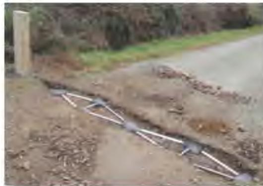
Installation Example with PYRO for Pedestrians and two ZELT Inductive Loops for Bicycles
