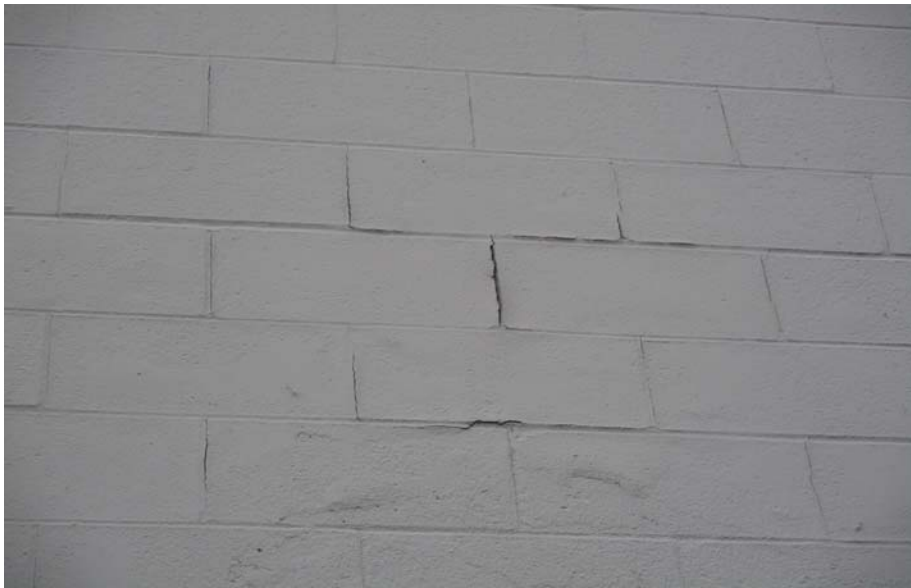
PHOTOGRAPH 1.4: A Pod - B2010
