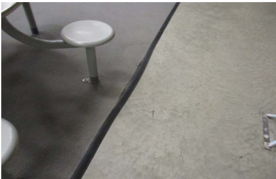
PHOTOGRAPH 1.14: A Pod - C3020
