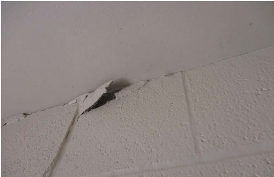
PHOTOGRAPH 1.10: A Pod - C1010
