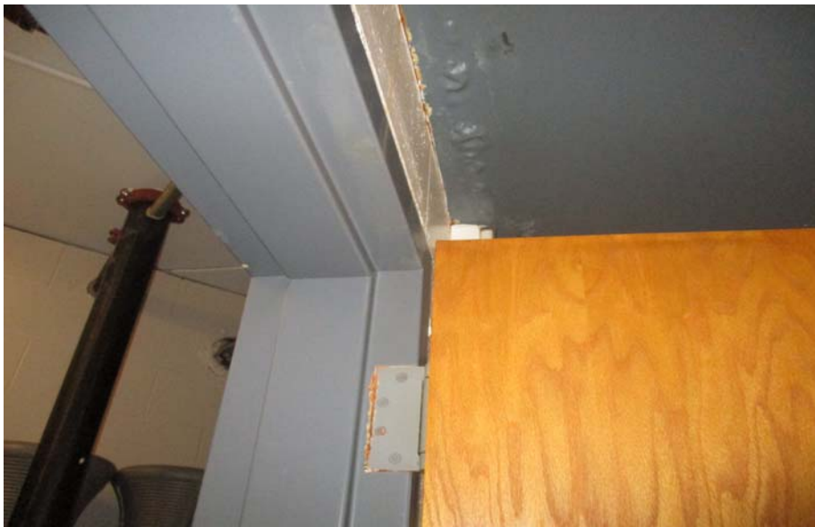
PHOTOGRAPH 1.8: A Pod - B3010
