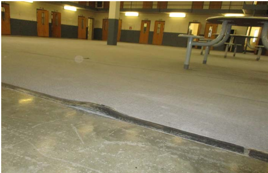
PHOTOGRAPH 1.13: A Pod - C3020
