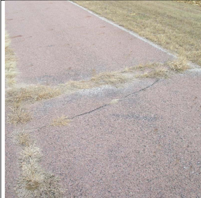
Photograph No. 11 24-foot perimeter road
