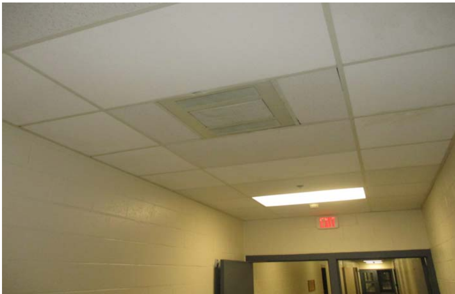
PHOTOGRAPH 1.17: A Pod - C3030
