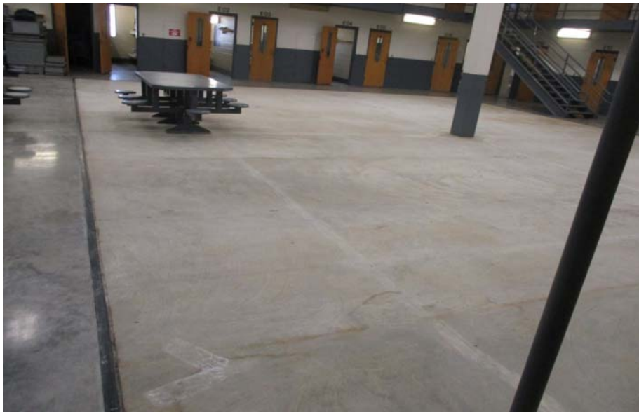
PHOTOGRAPH 1.16: A Pod - C3020
