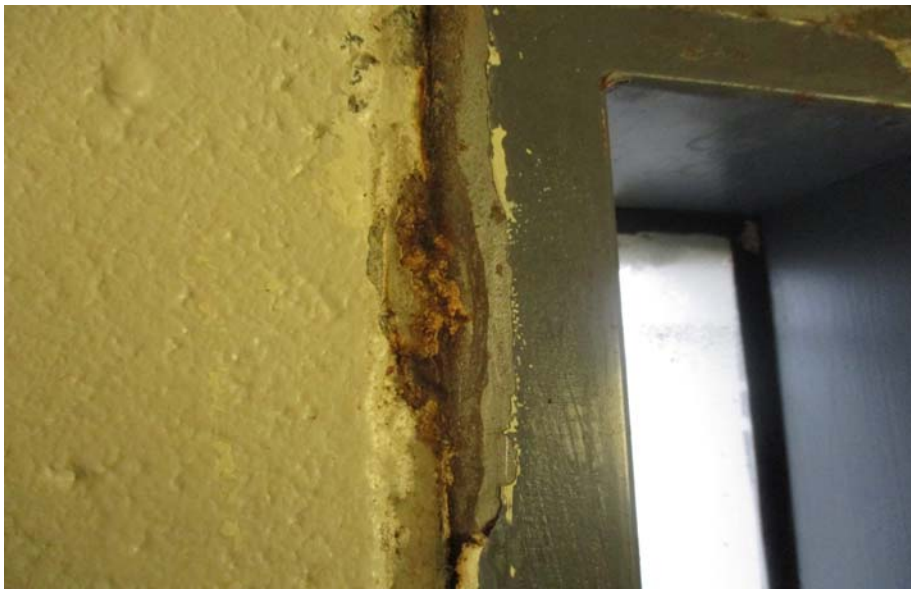
PHOTOGRAPH 1.5: A Pod - B2020
