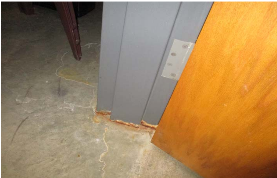
PHOTOGRAPH 1.12: A Pod - C1020
