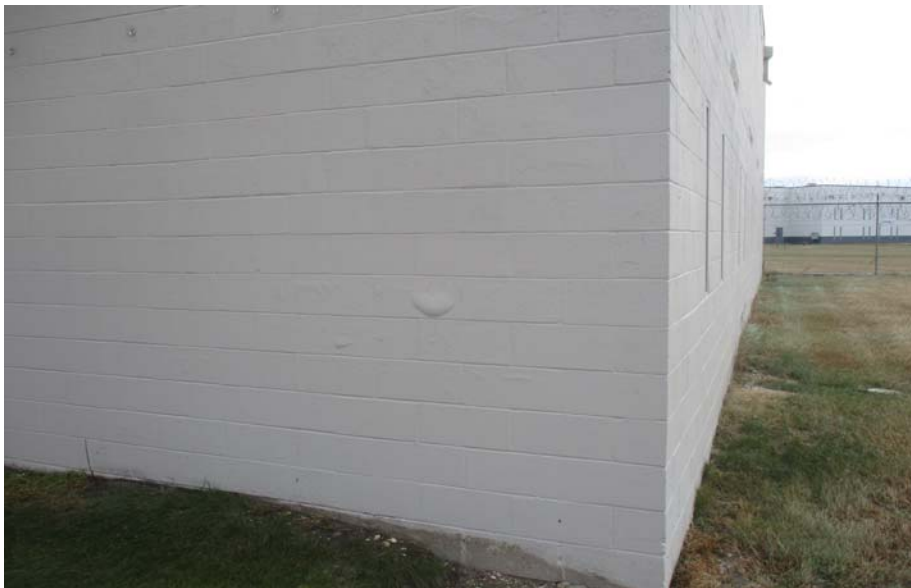
PHOTOGRAPH 1.3: A Pod - B2010
