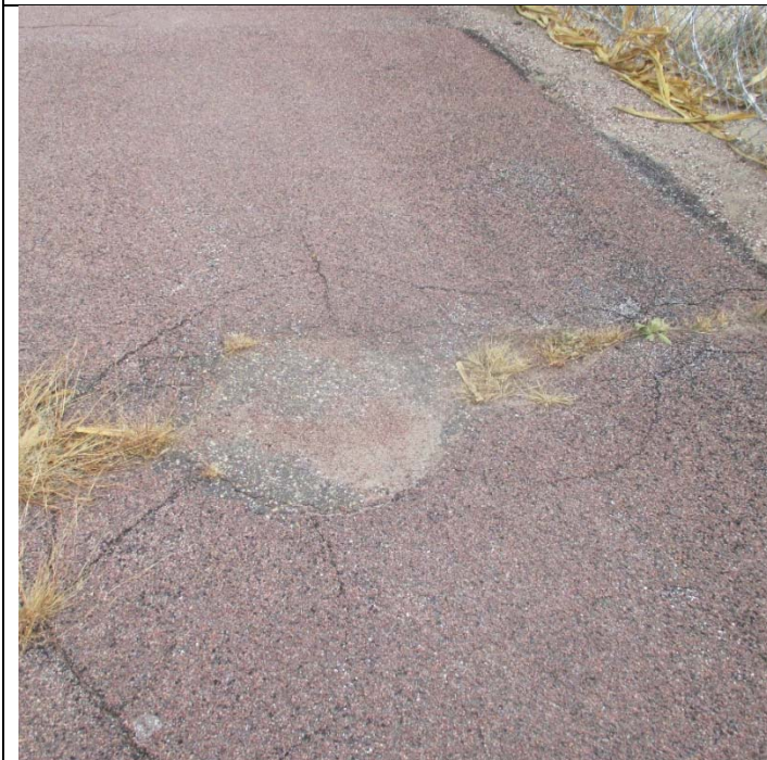
Photograph No. 10 Pothole on 15-foot perimeter road close to guard tower
