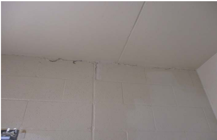
PHOTOGRAPH 1.9: A Pod - C1010
