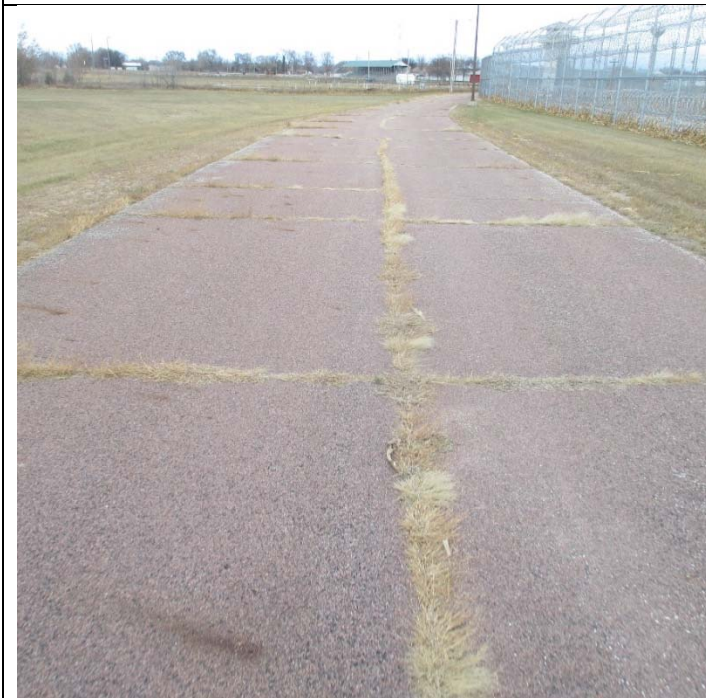
Photograph No. 12 24-foot perimeter road
