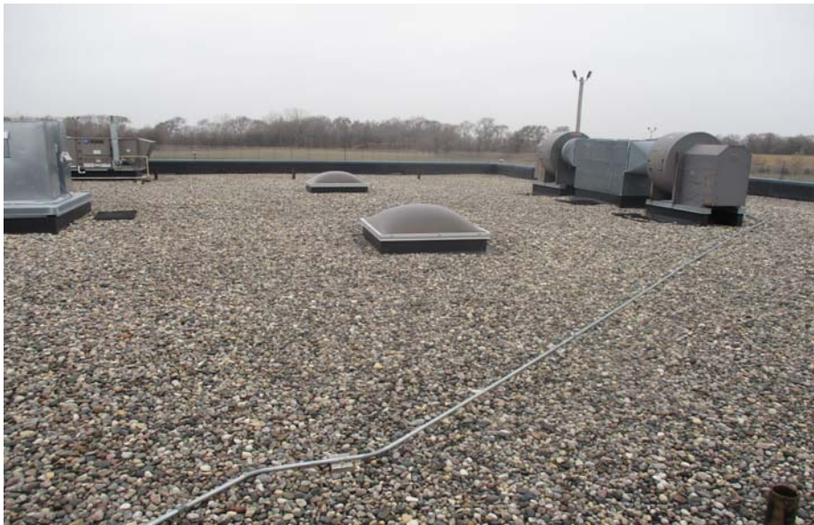
PHOTOGRAPH 1.7: A Pod - B3010
