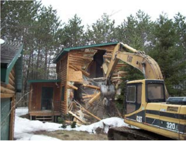
Removal of Flood Damaged Structure in Pine County Photo Courtesy of Pine County
