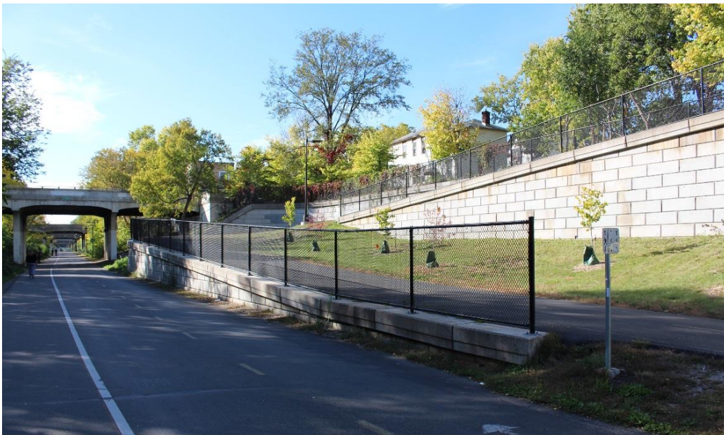
Figure 22. One of seven access ramps from the street into the trench; this one is located between 17 th and 18 th Avenues. Access ramps like this one extend the length of the block and take up approximately one-third of the trench width. Additionally, the concrete block construction of the access ramp create a new trench wall where there was none historically. Mead & Hunt, 2015.
