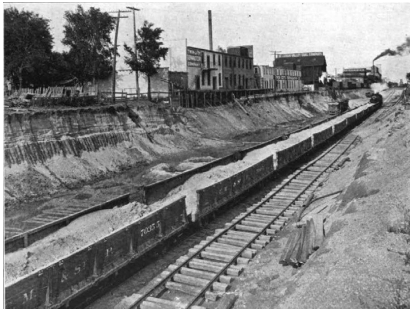
Figure 3. c.1915 photograph of the CM&StP Grade Separation under construction between Dupont and Emerson Avenues. Image from "Track Depression Work of the C.M. & St. P. Ry. at Minneapolis," Railway Review, July 17, 1915, pg. 70.
