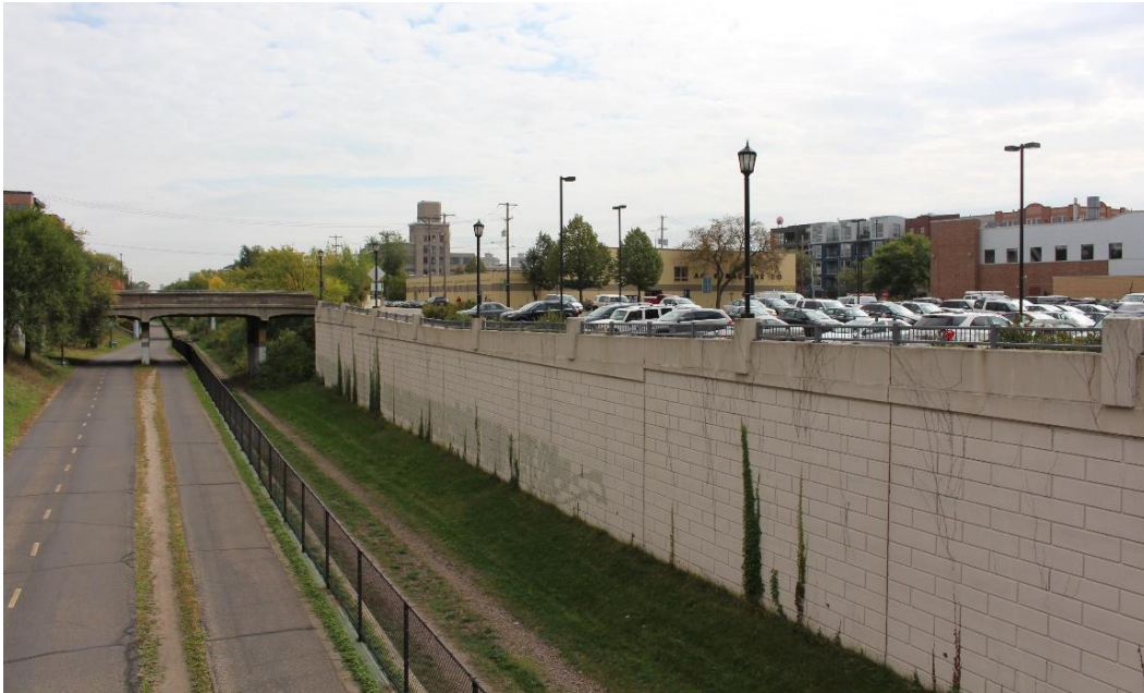
Figure 28. Example of a new trench retaining wall where none was historically, located between Hennepin and Freemont Avenues. Mead & Hunt, 2015.
