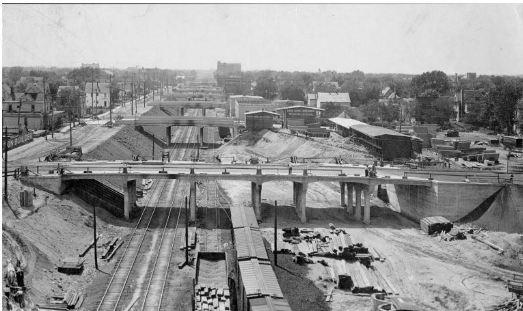
Figure 5. c.1915 photograph showing construction of 29 th Street, bridges over the CM&StP Grade Separation, and the rail yard at Clinton Avenue. The Clinton Avenue Bridge is in the foreground followed by the 3 rd , 2 nd , and Stevens Avenue Bridges (all of which are nonextant). Photograph by C.J. Hibbard, c.1915, Minnesota Historical Society.
