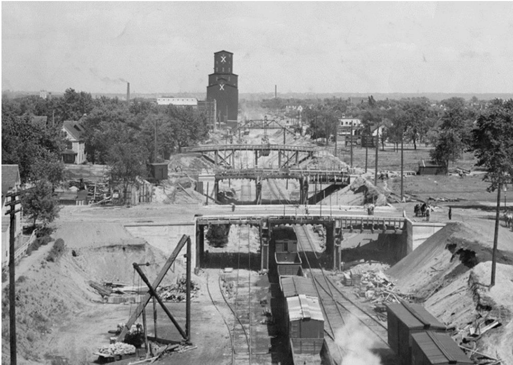
Figure 2. c.1915 image of the grade separation under construction. View from 5 th Avenue east toward Portland and Oakland Avenues. Note the Bagley Grain Elevator (later to be replaced by the Stewart Grain Elevator; nonextant) in the background. Photograph by C.J. Hibbard, c.1915, Minnesota Historical Society.
