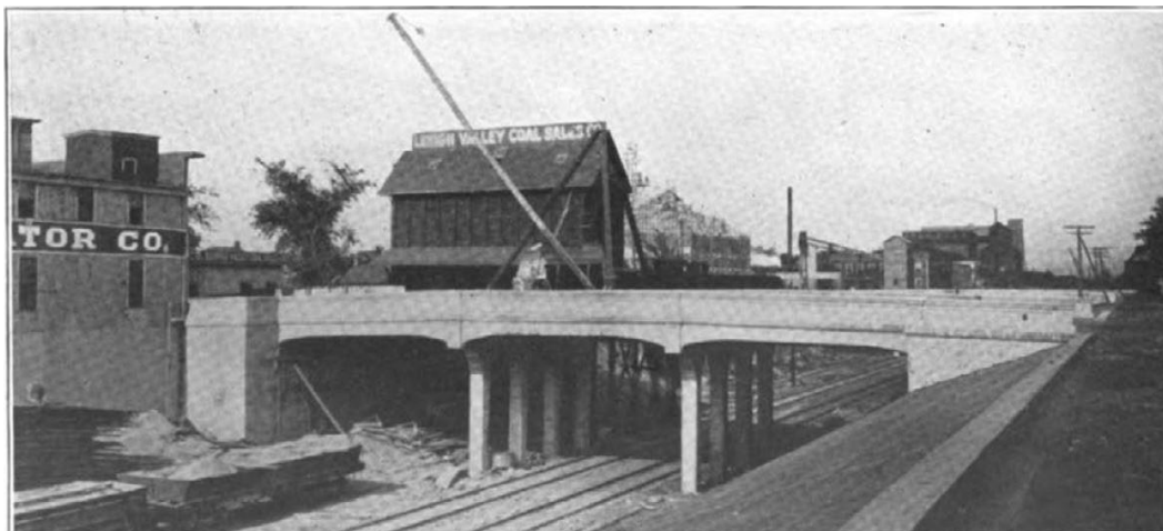
Figure 11. The Colfax Bridge after construction. Note the industrial building on the far right that serves as the embankment wall. Image from "Track Depression Work of the C.M. & St. P. Ry. at Minneapolis," Railway Review , July 17, 1915, 72.
