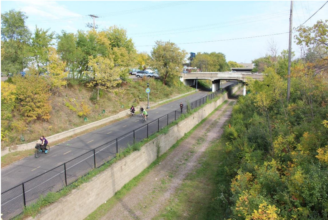
Figure 21. Elevated trail between Nicollet and Stevens Avenues. The use of a retaining wall to elevate the trail significantly alters the original grade of the rail corridor. Mead & Hunt, 2015.
