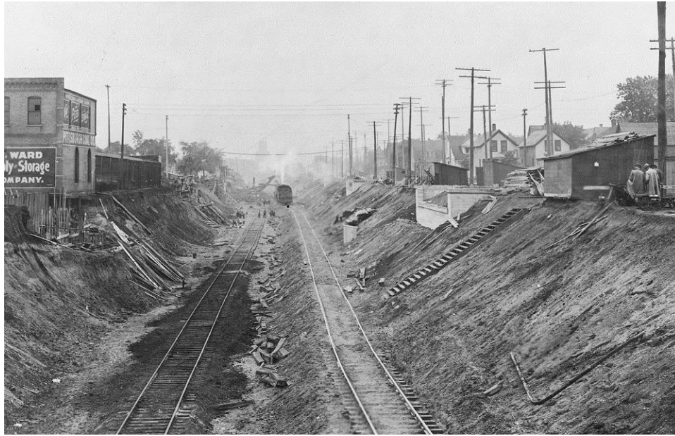
Figure 1. Grade separation trench under construction, view looking west from 1 st Avenue (now the location of I-35W). Note bridge abutments under construction. Image from the City of Minneapolis Transportation Department photograph collection, courtesy of Gemini Research. 3
