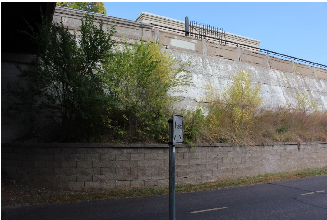
Figure 7. An original trench embankment retaining wall with original concrete parapet in the background and a new ashlar block retaining wall in the foreground, located between Pleasant and Nicollet Avenues. Mead & Hunt, 2015.
