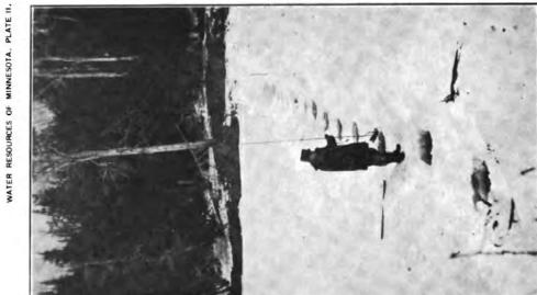
A. DISCHARGE MEASUREMENT OF VERMILION RIVER BY MEANS OF CAR AND CABLE.
