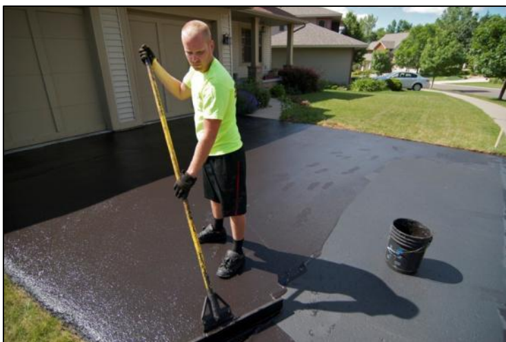
Figure 3-38. Asphalt-based sealants are a suitable alternative to CT-sealants, shown here being applied to an asphalt driveway.
