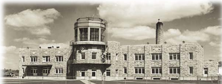
St. Paul Downtown Airport Terminal Building – Year 1939
