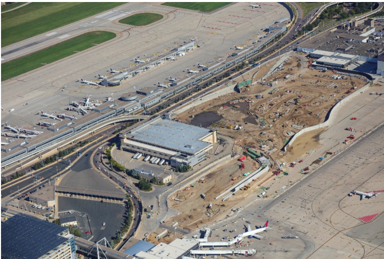
Construction Progress on the Terminal 1-Lindbergh Silver Parking Ramp
