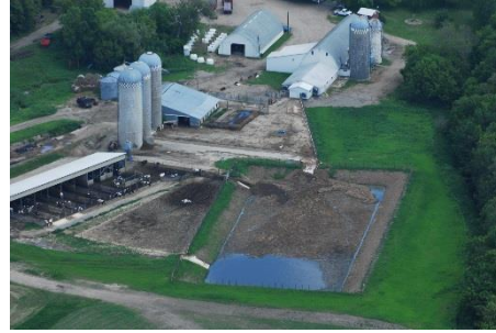
Figure 12. Manure treatment system in Stearns County.
