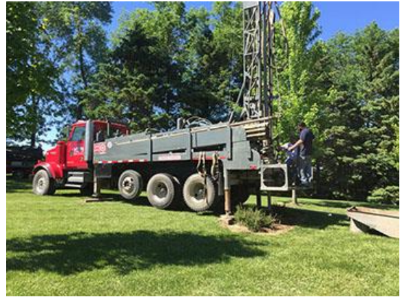
Figure 27. Typical well drilling installation.
