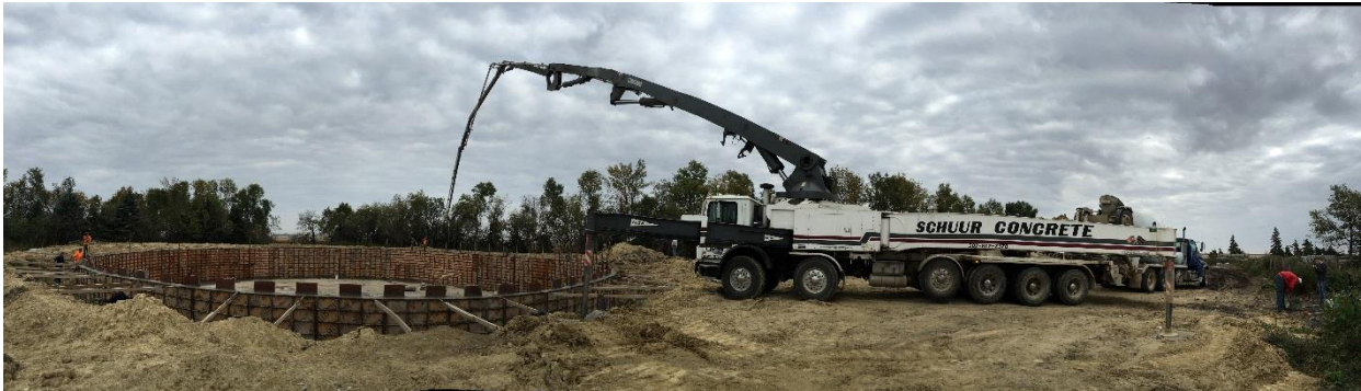
Figure 13. Installation of manure storage structure in Olmsted County.
