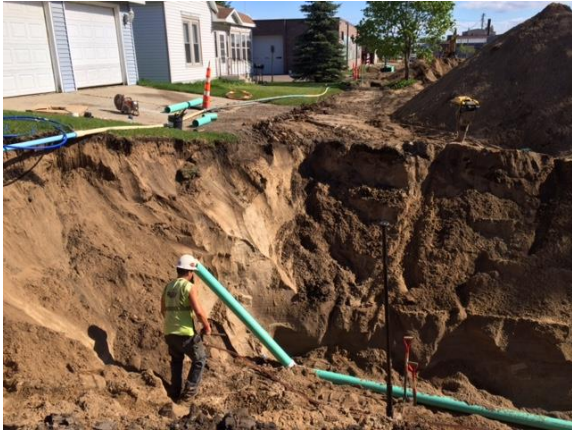
Figure 23. Connecting private lateral lines to municipal system, Wadena County.
