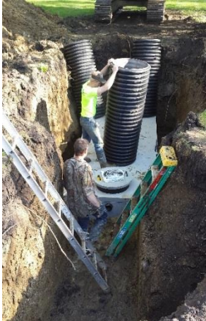
Figure 22. Installation of a typical septic tank and mound drain field, Watonwan County.
