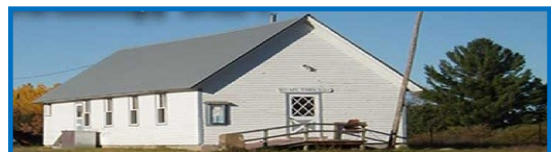
Wilma Townhall in Pine County received broadband equipment to develop a hot spot at their town hall.
