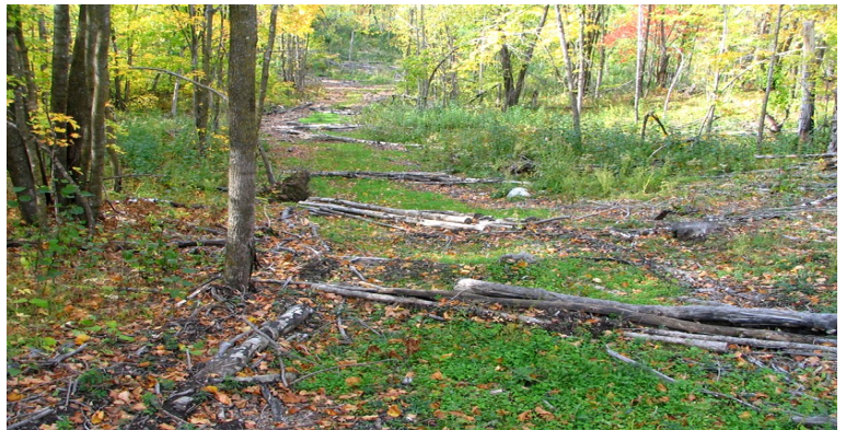
Use of erosion control measures, such as these log water bars, following harvesting is a key forest management guideline used to minimize impacts to water quality .
