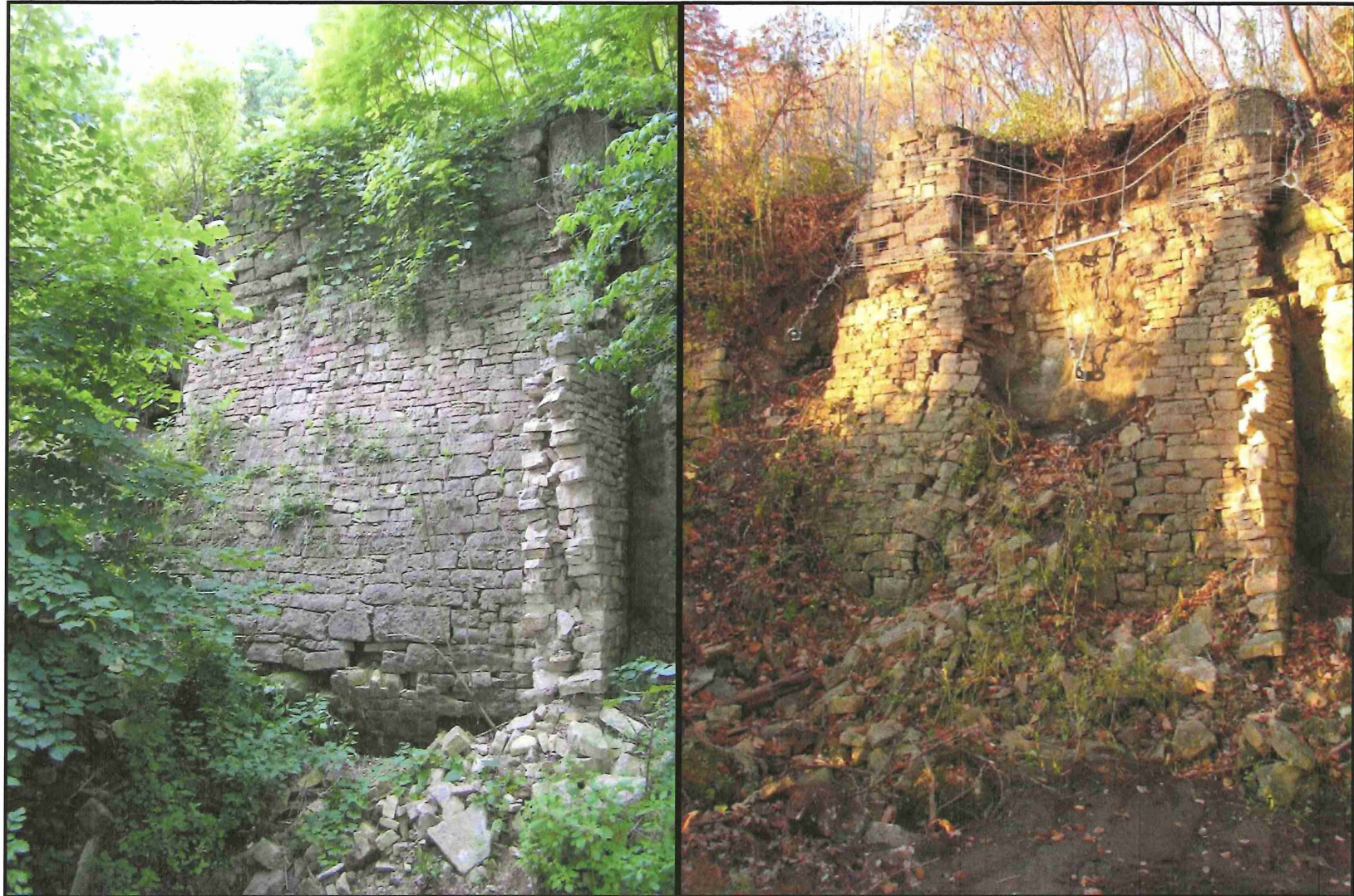
FIGURE 8. WALL D AS IT APPEARED IN 2004 (LEFT) AND AFTER STABILIZATION IN 2015 (RIGHT), VIEW TO SOUTHWEST
