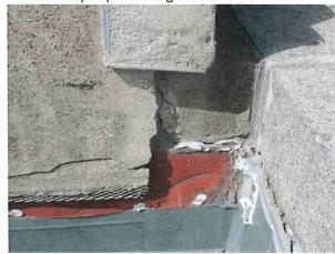
View of ductwork brackets and failing parapet joints
