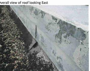
View of failing parapet flashing seam and finish
