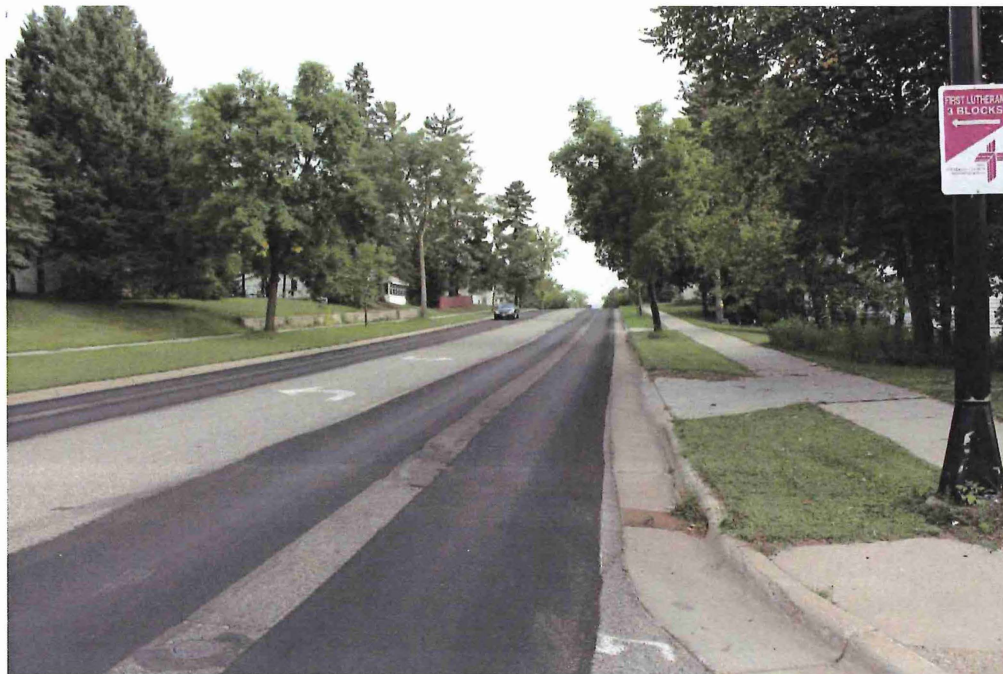
Figure 10. TH 38 in Grand Rapids. Note the wide roadway, center turn lane, and curb and gutter. Historically the center turn lane was a paved median. Mead & Hunt, 2015.
