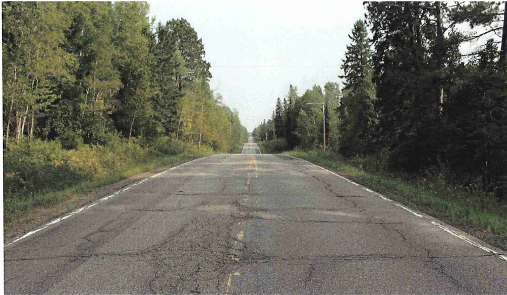
Figure 4. TH 38 within the Chippewa National Forest boundaries. Note the narrow gravel shoulder. Mead & Hunt, 2015.
