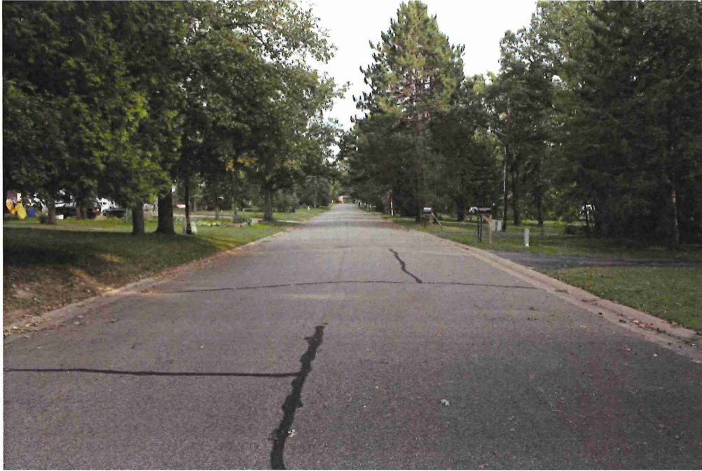
Figure 21. Former alignment of SR 1, now Audrey Lane. Note the width, bituminous surfacing, and curb and gutter. Mead & Hunt, 2015.
