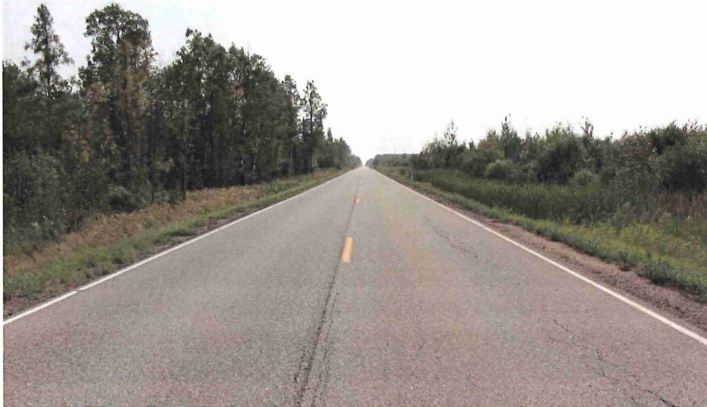
Figure 6. TH 38 near Effie. Note the continued use of graveled shoulders here and flatter topography. Mead & Hunt, 2015.
