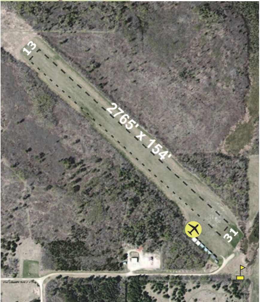
Remer Municipal Airport
