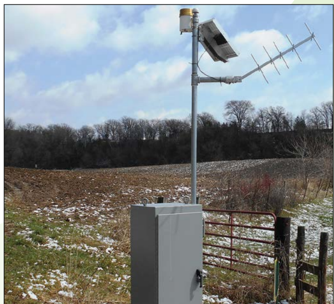
River gauge for Whitewater State Park.
