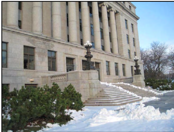
Exterior Stairs - Missing Handrails - Monumental Steps
