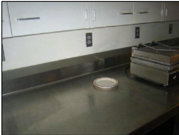
Branch Wiring - Outlets in Kitchen Not GFCI Type
