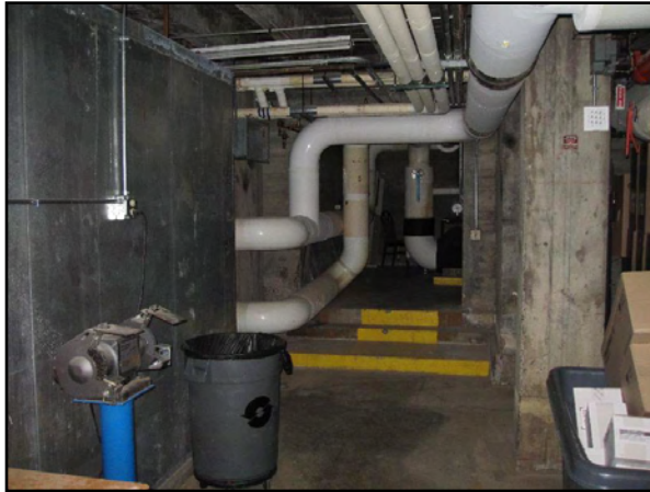
Four Pipe Distribution System w/Pump Renewal
