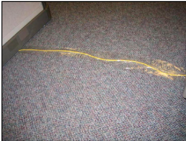
Communication Wiring - Improperly Installed - Corridor 180B
