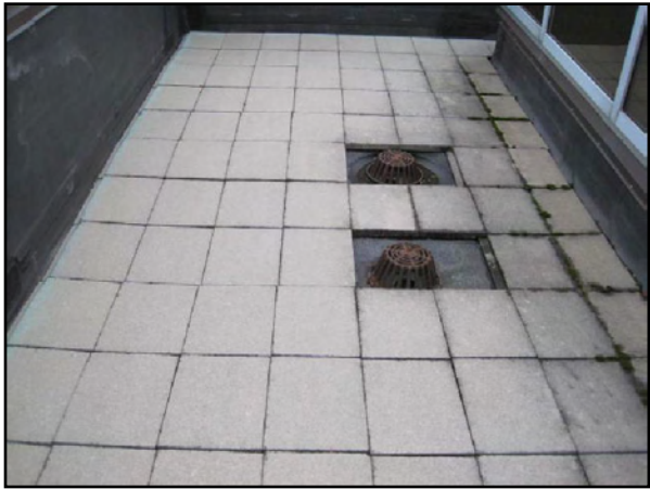
Single-Ply EPDM with Pavers on Roof - 1985 Renewal Single-Ply EPDM with Pavers on Roof - 1985 Renewal
