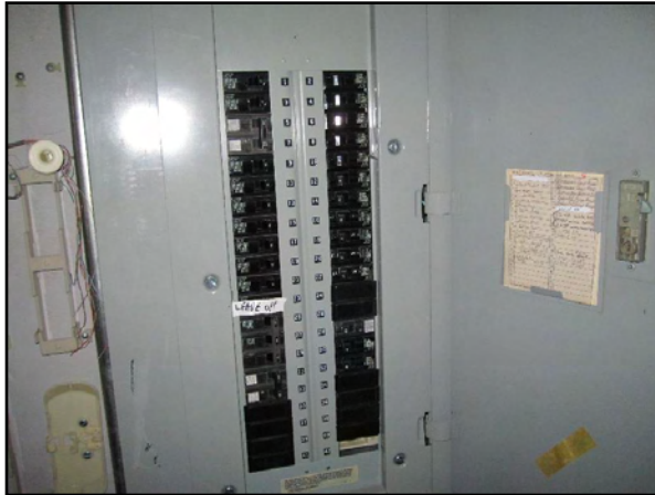
Emergency Panelboards - Approaching Rated Life
