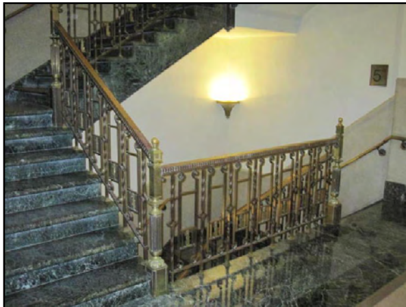
Guardrails - Non-Compliant Heights - Monumental Stairs
