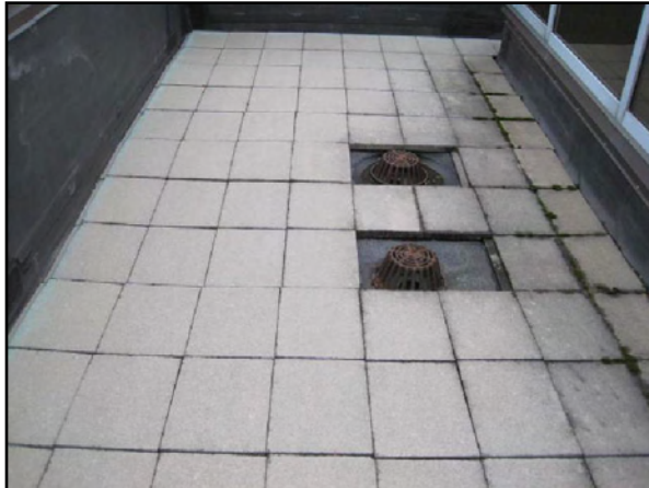
Single-Ply EPDM with Pavers on Roof - 1985 Renewal
