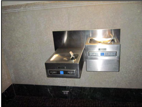
Water Coolers - Wall-Mount Dual-Height Renewal
