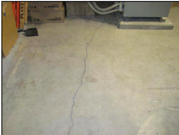
Substructure - Basement Slab Cracks
