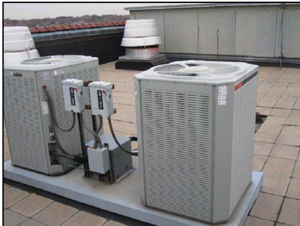
Branch Wiring – Outlets Not Installed at HVAC Units
