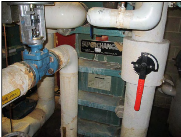
Heat Exchanger - Liquid/Liquid - Plate and Frame Renewal
