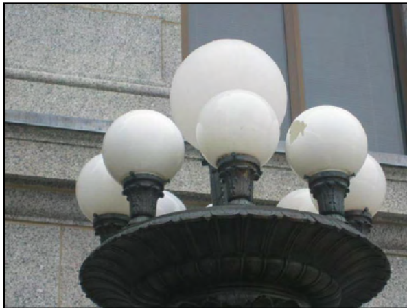
Exterior Lighting - Luminaires in Disrepair
