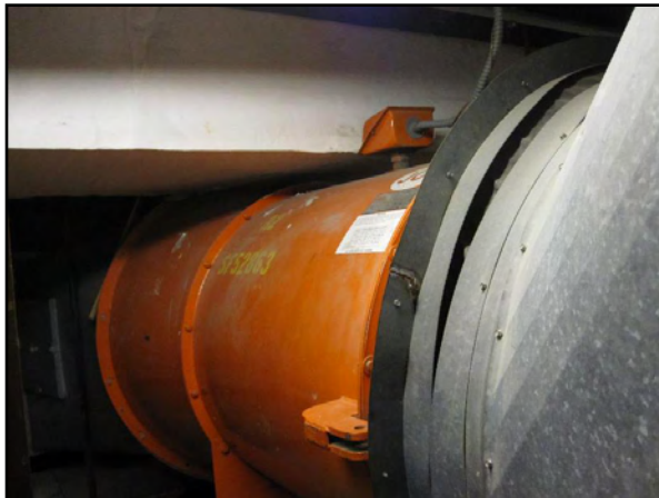
Exhaust System - General Building - In-Line Renewal
