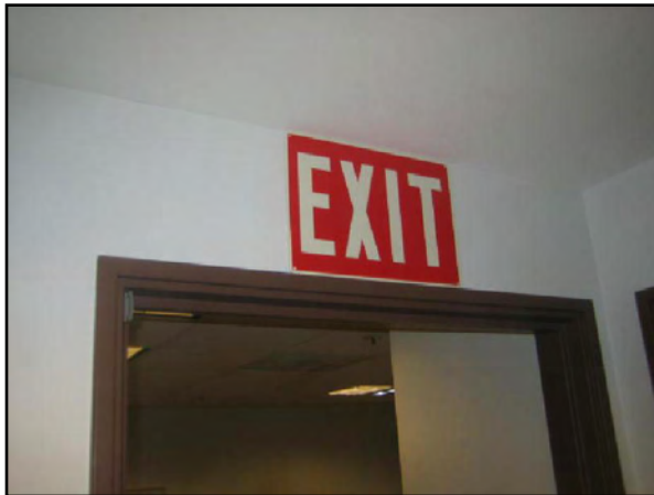
Exit Signs – Not Properly Illuminated
