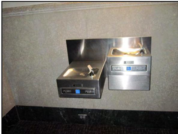
Water Coolers - Wall-Mount Dual-Height Renewal
