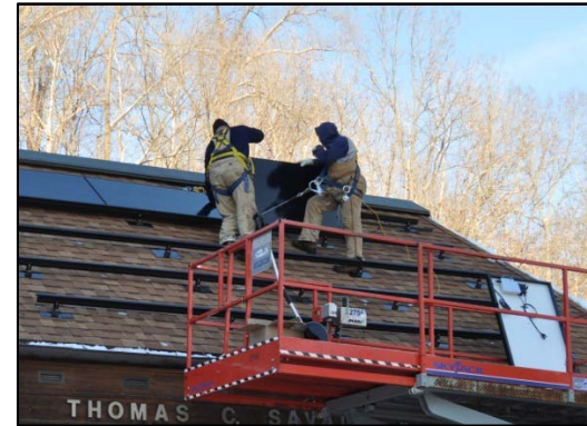
Solar panel installation at Ft. Snelling State Park
