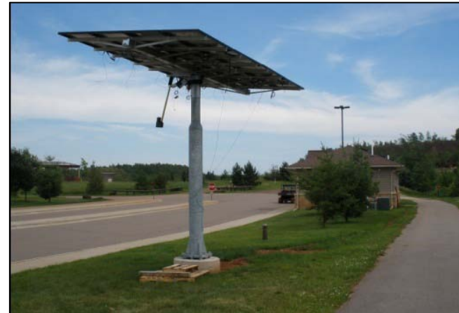
One of the three solar arrays at the Iron Range OHV
