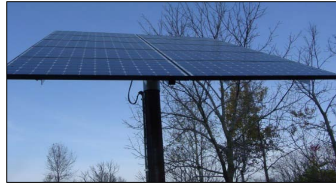
One of the two solar arrays at Great River Bluffs State Park
