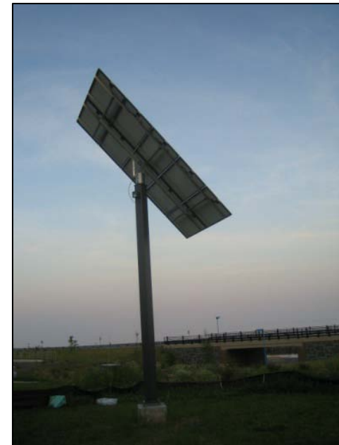
Solar array at McQuade Small Craft Harbor
