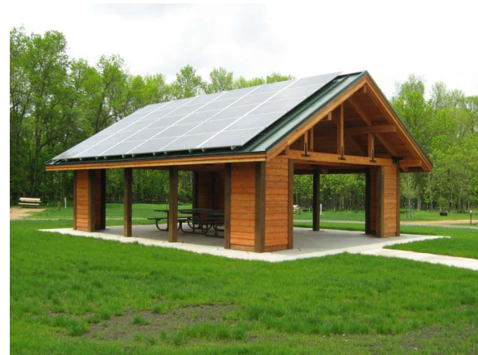
Picnic shelter with roof mounted solar panels at Lake Shetek State Park
