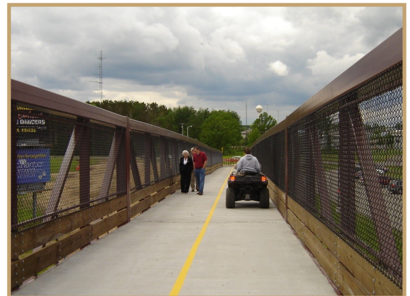
Pedestrian bridge over TH 169 at Onamia
