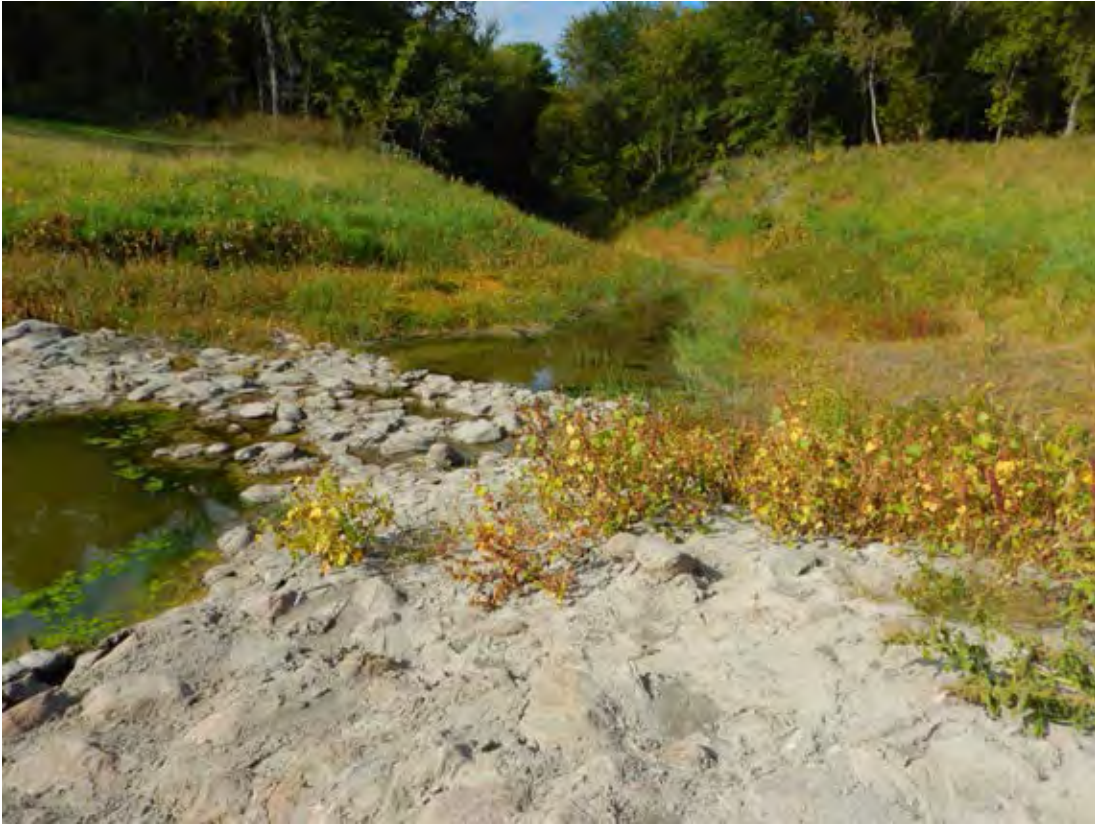
CC Photo 5: Immediately downstream of upper grade control structure.
