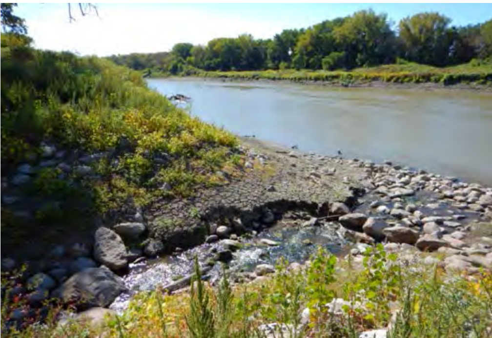
SR Photo 38: Outlet to Red River. Sediment above constructed rock outlet assumed to be material deposited by Red River Floods in spring and scoured by Grand Marais Creek after coming on-line. Note change in water clarity between Grand Marais Creek and Red River at confluence.
