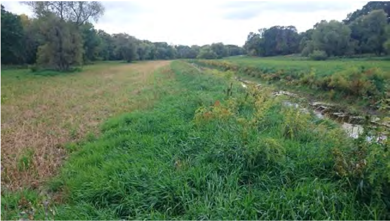
SR Photo 4: East bank immediately downstream of Diversion Structure.
