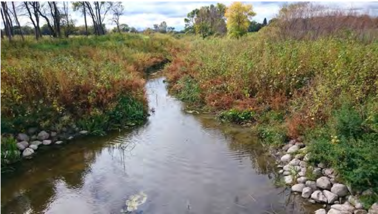
SR Photo 33: Rocked channel border above Boulder Vane.
