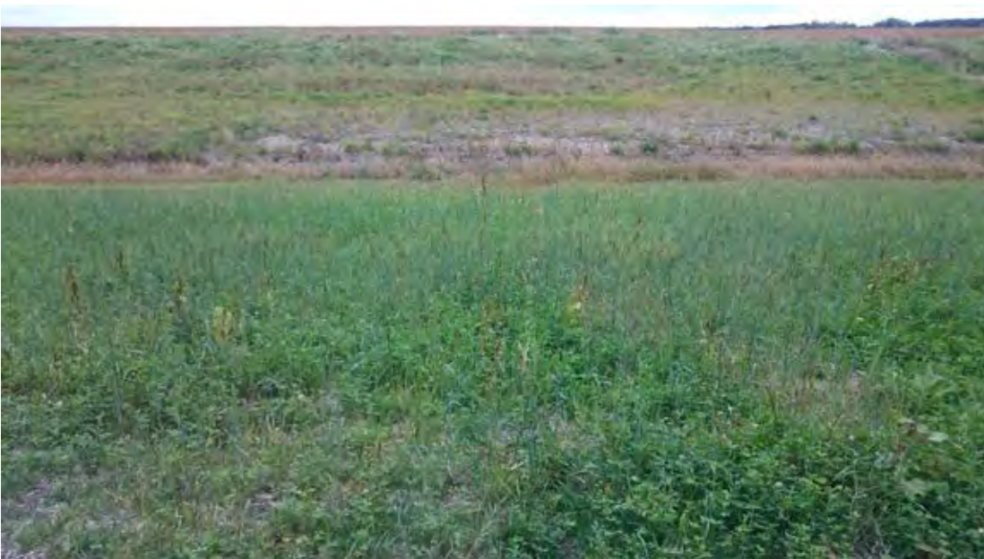
CC Photo 2: Stabilized slopes along upper channel. Note erosion at lower elevations near water level.
