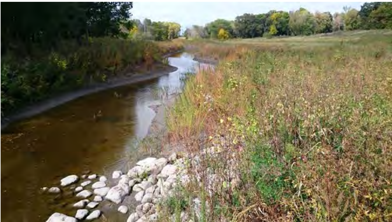
SR Photo 23: Riffle Boulder Vane below railroad car bridge.
