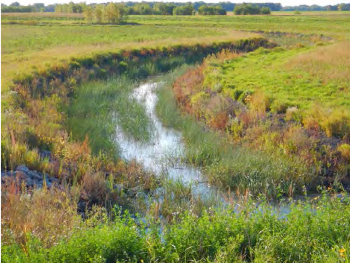
SR Photo 9: Constructed channel looking west from 470th Avenue NW. Channel dominated by Softstem Bulrush.
