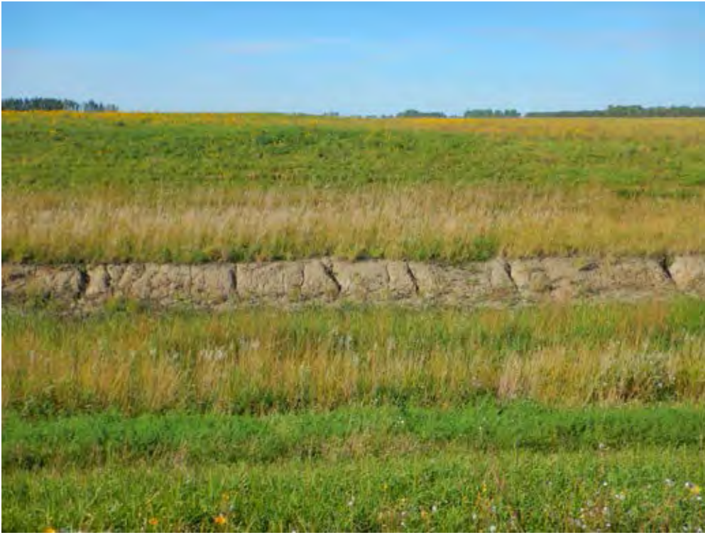
SR Photo 7: Constructed channel. Above
