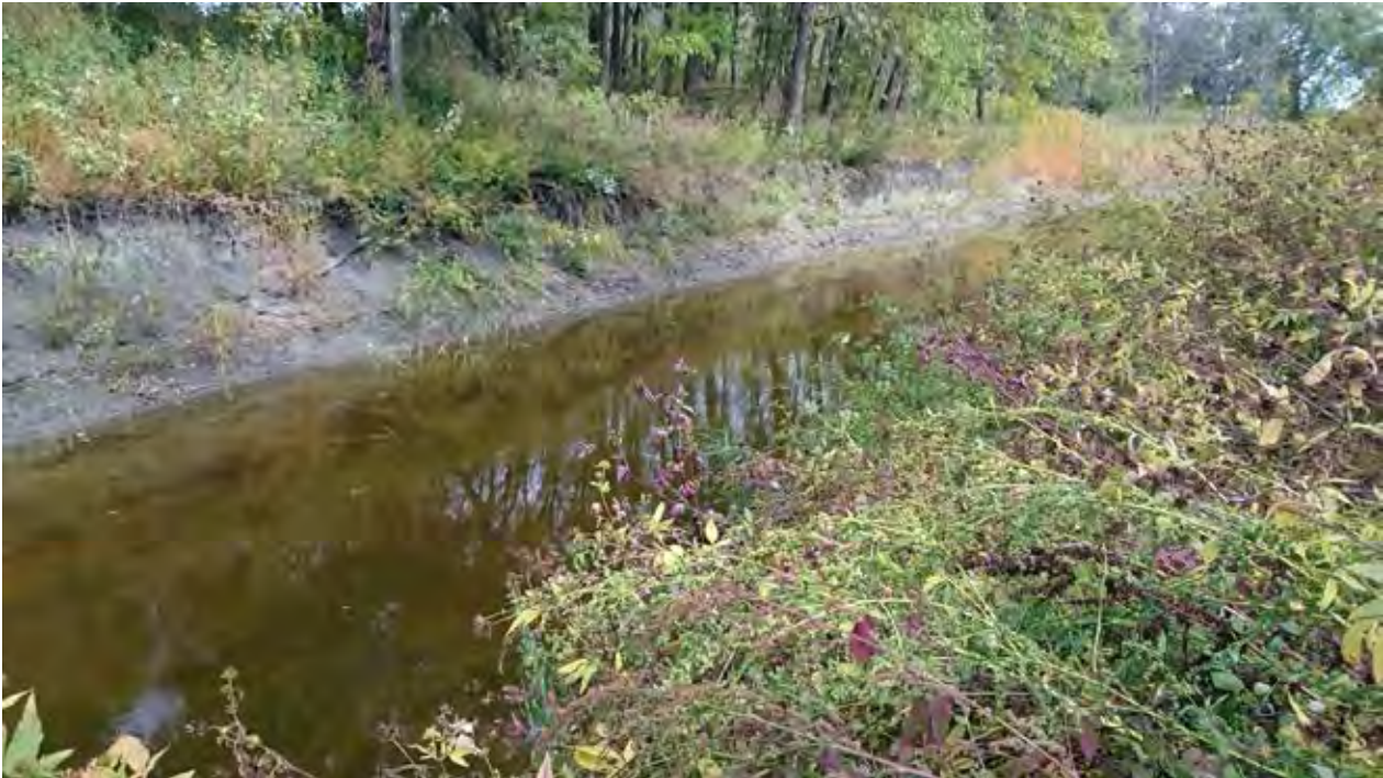
SR Photo 25: Exposed banks where channel was excavated in forested areas.
