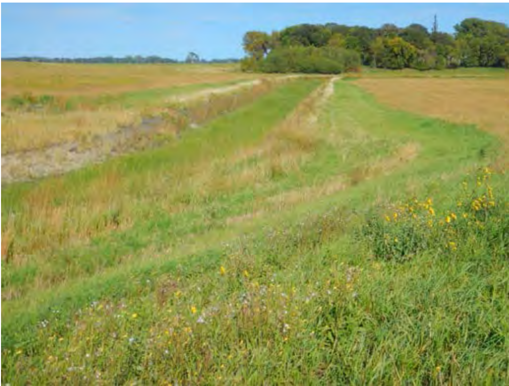
SR Photo 6: Constructed Channel. Upper areas seeded to “Special Seed Mix.” Lower slopes not seeded, channel dominated by Hybrid Cattail.
