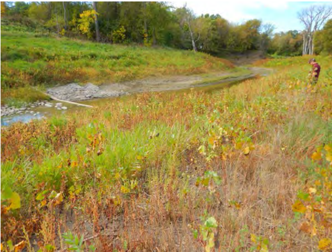
CC Photo 8: Lower grade control structure with upland grassland.
