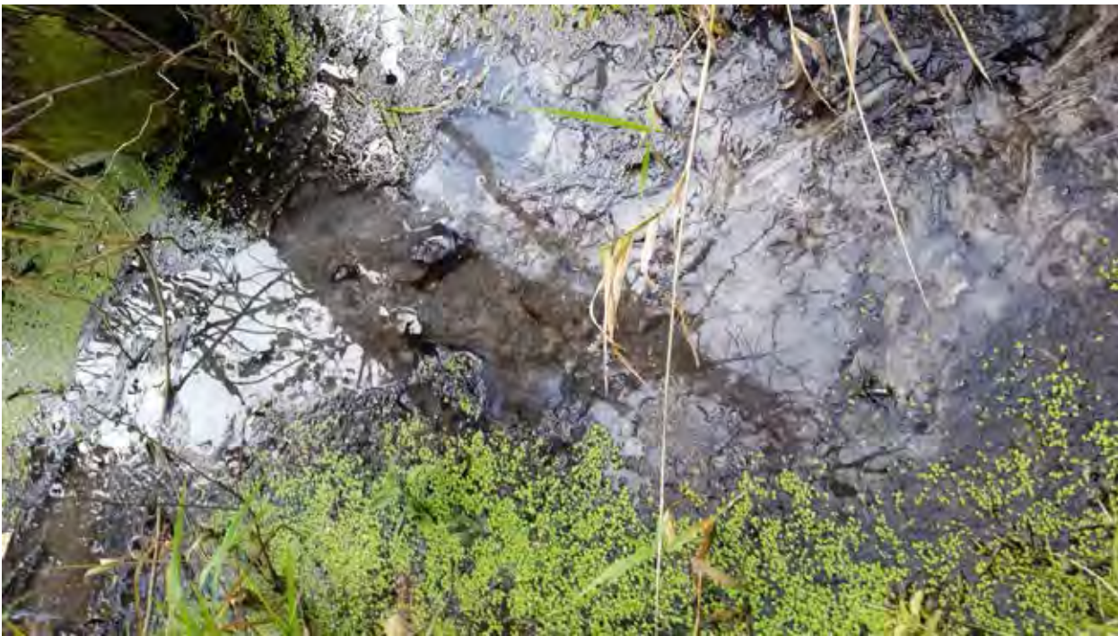
Figure 9 - Calcareous seepage at GPS point 476
