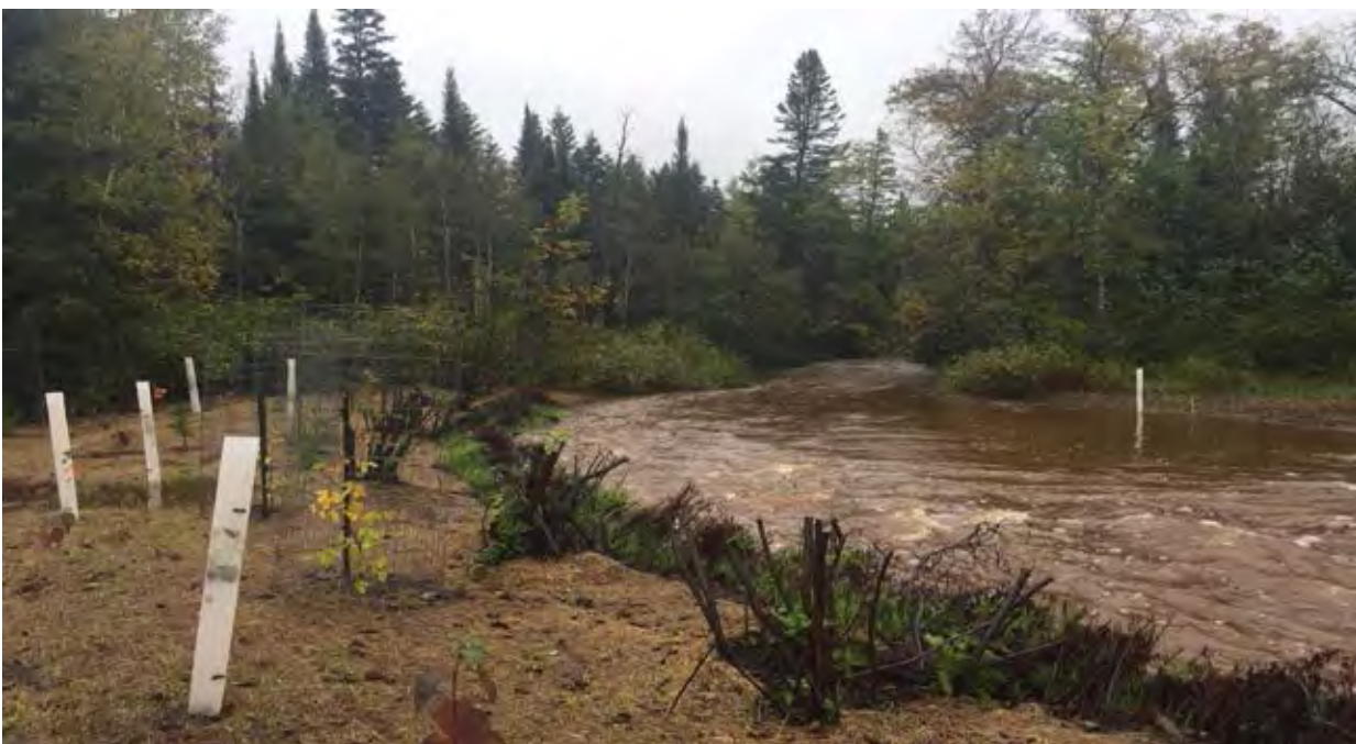
Figure 4 - Representative image of toe wood (near bank) and onsite transplants (near bank) along with the tree and shrub plantings with browse protection.
