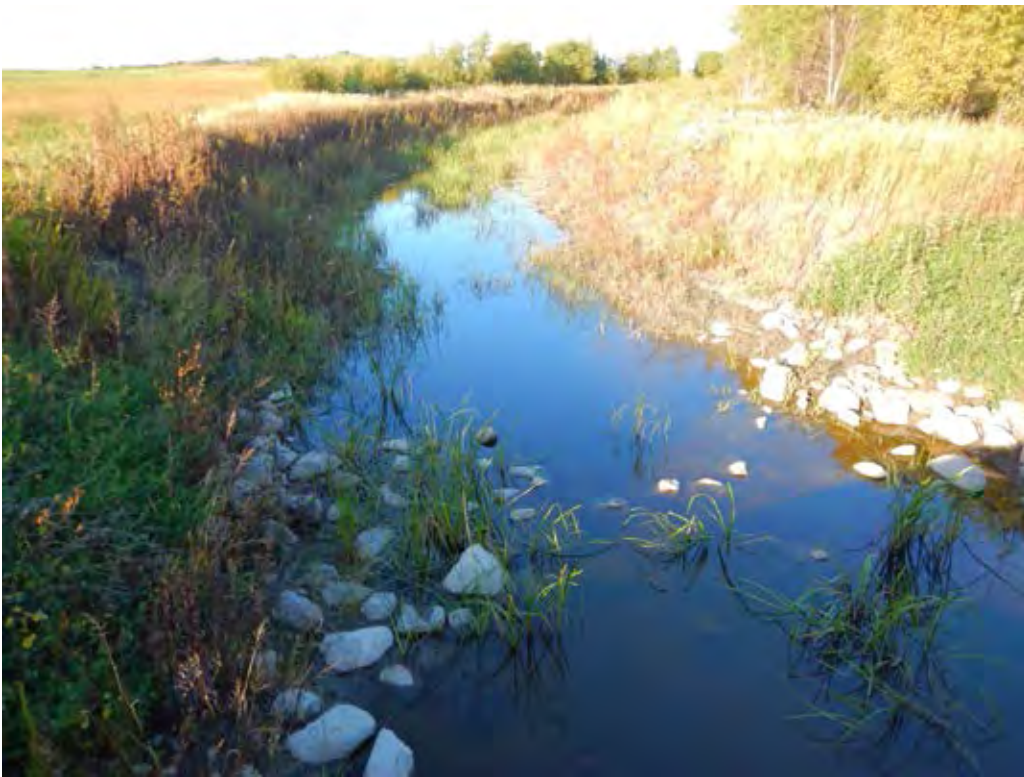
SR Photo 12: Ellipse Channel Riffle at 171+25. Vegetation is volunteer.
