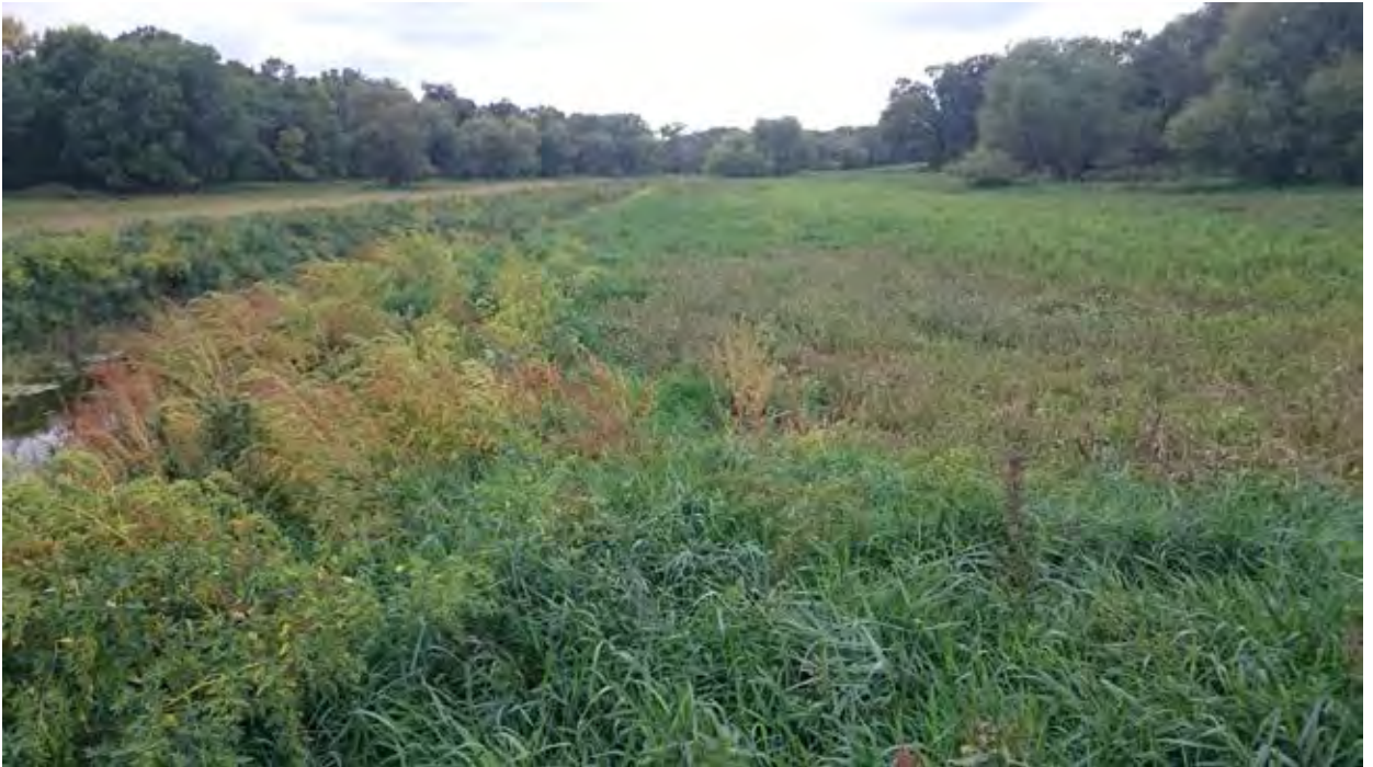
SR Photo 5: West bank immediately downstream of Diversion Structure.
