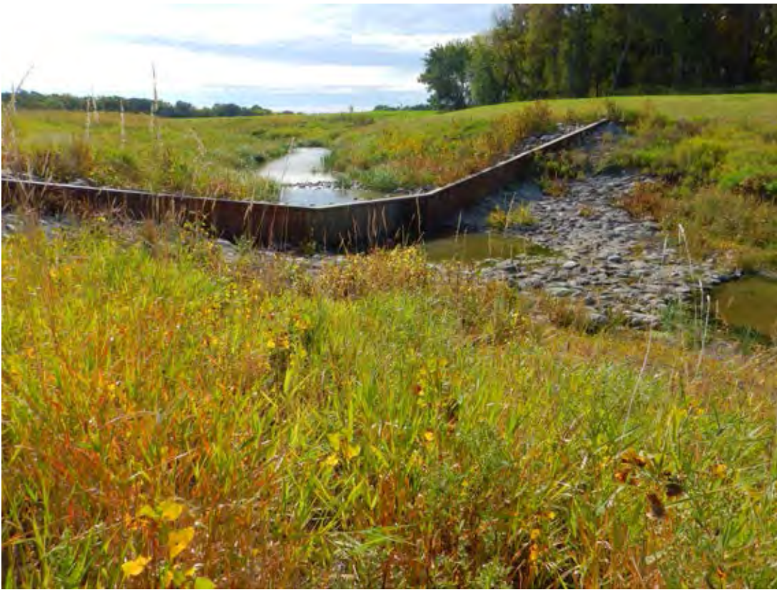
CC Photo 4: Upper grade control structure.
