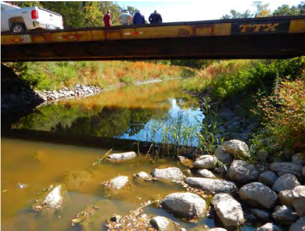
SR Photo 27: Railroad car bridge with Boulder Vane in channel below.
