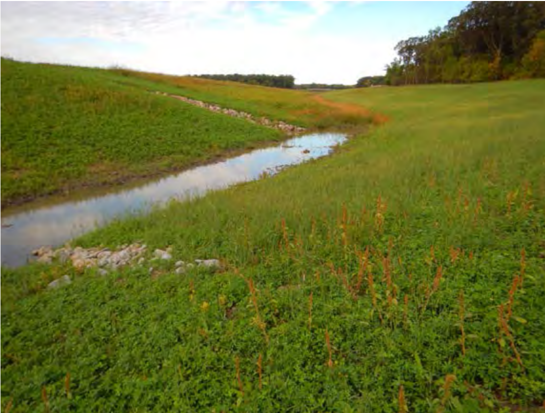
CC Photo 1: Stabilized slopes immediately south of Diversion Structure.
