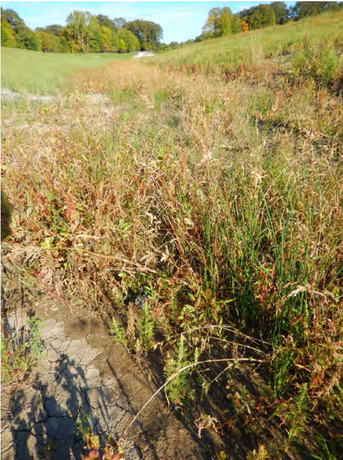
CC Photo 3: vegetation growing in the bottom of the cut channel.
