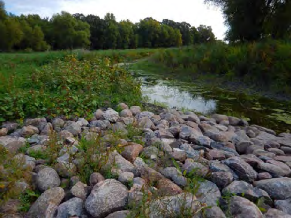
SR Photo 1: Grand Marais Creek at location of Diversion Structure.
