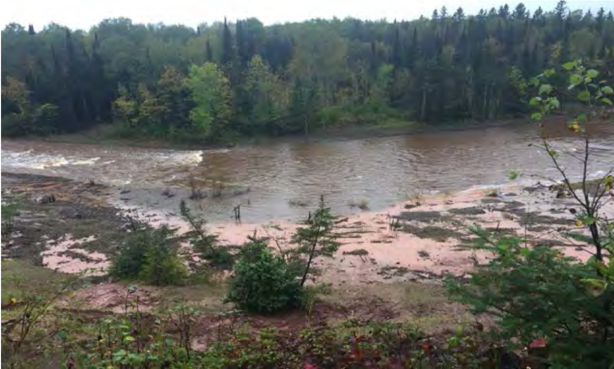
Figure 5 - Representative image of stabilization (bankfull bench). As illustrated in the photograph the created bankfull bench was appropriately being accessed (over-topped) by a near bankfull flow event.
