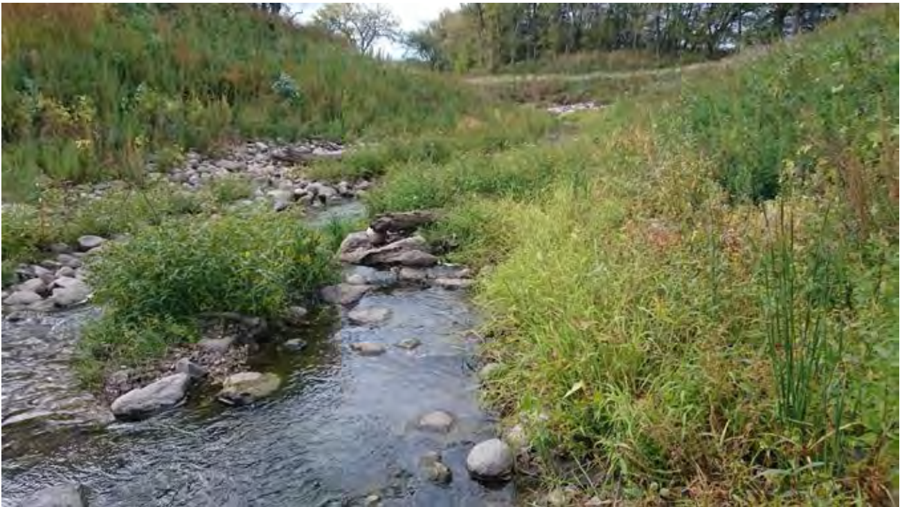
SR Photo 34: Entering the V Channel Riffle at downstream portion of project.
