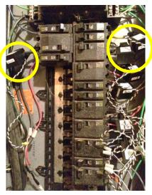
Figure 4. Current sensors snapped around different circuits within the circuit breaker panel
