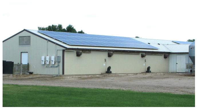
Picture 3. 27 kW Solar PV System on WCROC Swine Facility – West Side
