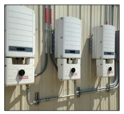
Figure 4: SolarEdge SE9K Three Phase Inverters on the WCROC Swine Barn.
