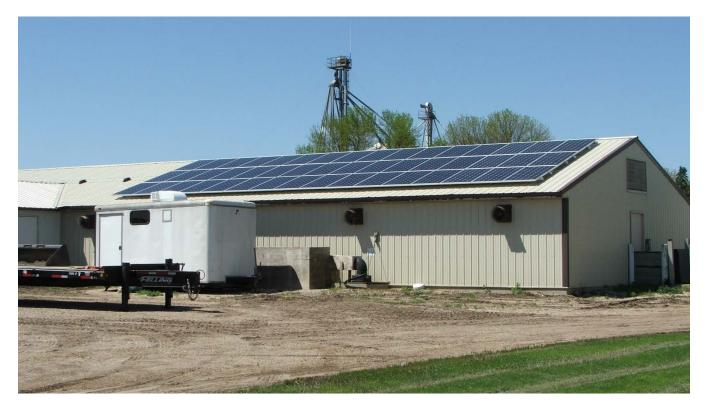
Picture 4. 27 kW Solar PV System on WCROC Swine Facility – East Side
