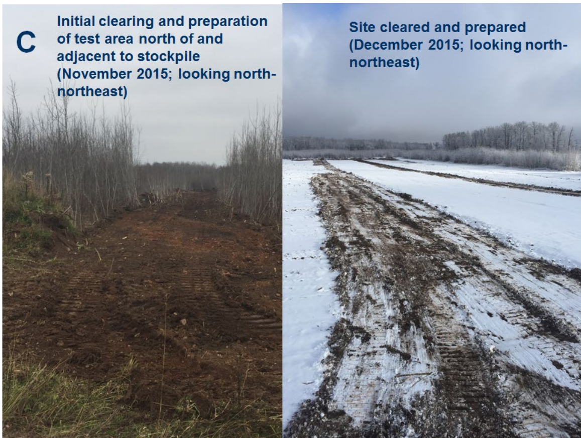
Figure C. Project site preparation.
