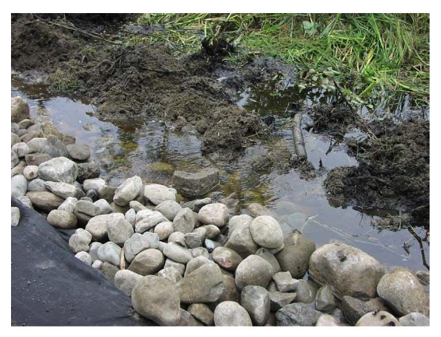
Figure 48. Downgradient of Wirt Road showing water flowing out of the porous roadbed.
