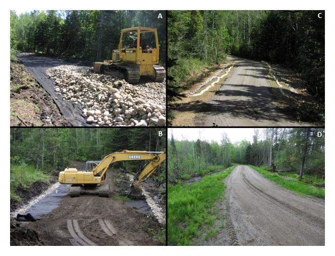
**Figure 40.** Sequence of Wirt road restoration: A) Roadbed was removed, then geotextile was laid out and 12" of 4 to 6-inch rock was spread out over the fabric, B) then another layer of geotextile fabric and more dirt was laid over the top of the rock, C) additional rock was placed at the toe of the slope over the geotextile fabric exposed below the gravel roadbed and erosion blankets were placed to cover the disturbed surfaces alongside the road, D) finished road as of June 2017.
