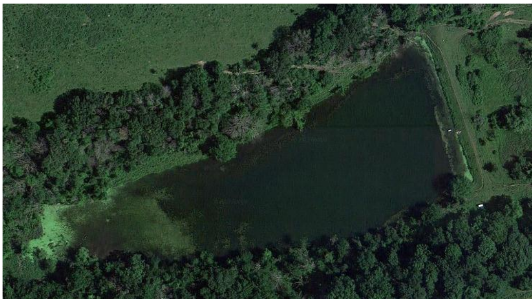
Figure 6. 5 acre surface area SCS Grade Stabilization Structure on un-named creek, Dodge Co., MN.
