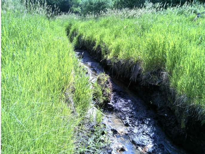
Unauthorized ditch dug by landowner on protected property showing significant erosion
